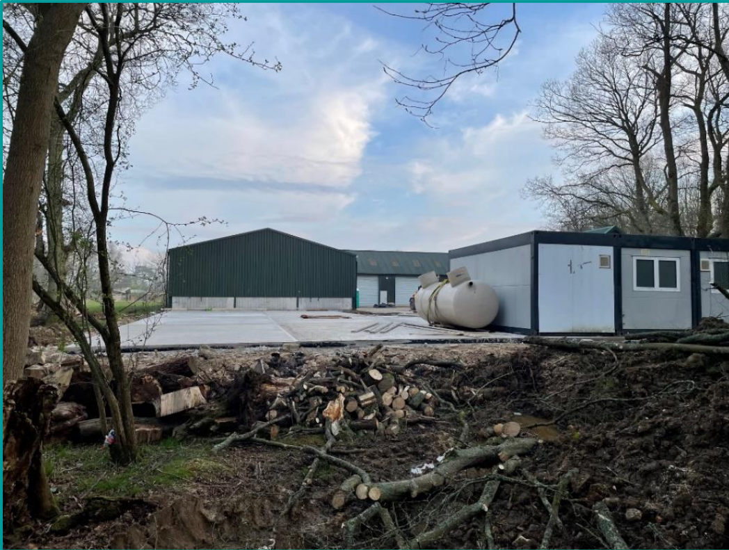
Tree removal and new hardsurfacing, including possible drainage or fuel tank
