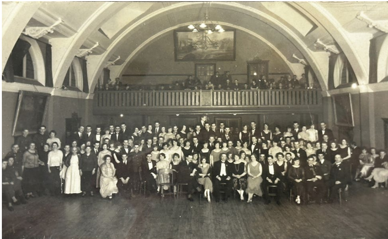
2.15 1920s photograph of the south end of the hall with dance participants on sprung dancefloor and the original balcony balustrade (Hitchin Museum, 12673.25, Box KI)
