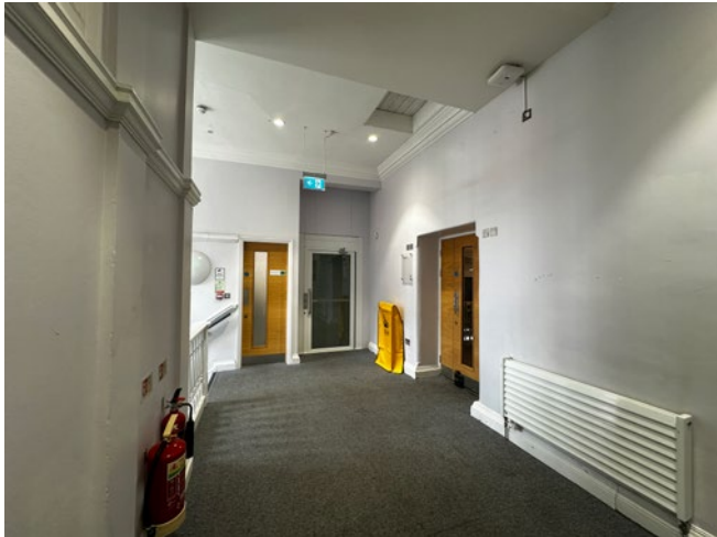
3.65 Looking north-west in F1
