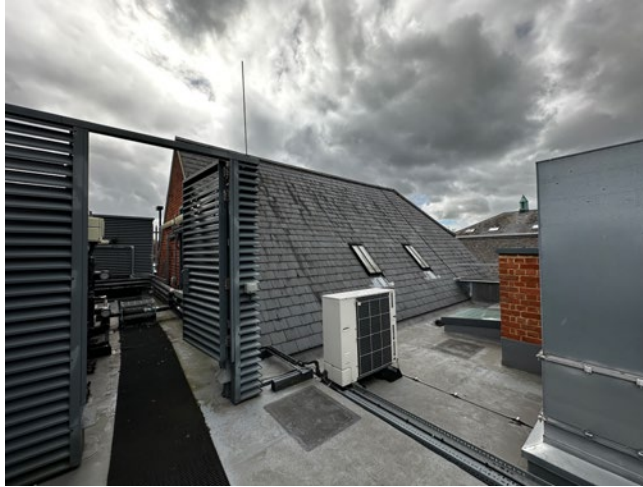
3.26 Looking east at the west pitch of the Workmen's Hall
