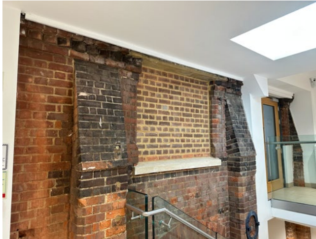
3.85 Looking east on second floor landing S1
