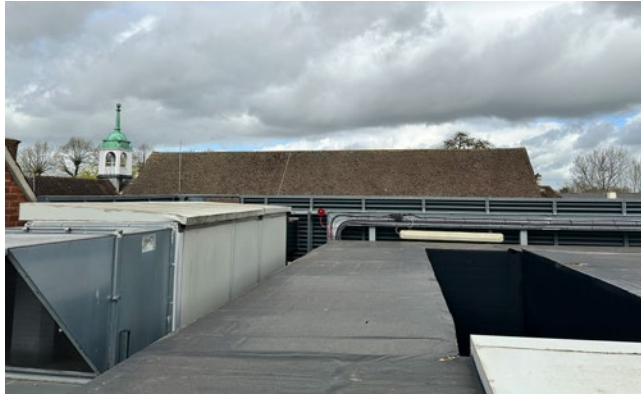
3.22 Town Hall roof seen across modern former gym flat roof
