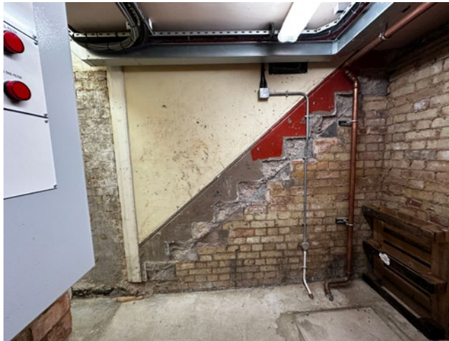
3.35 South wall of B6
