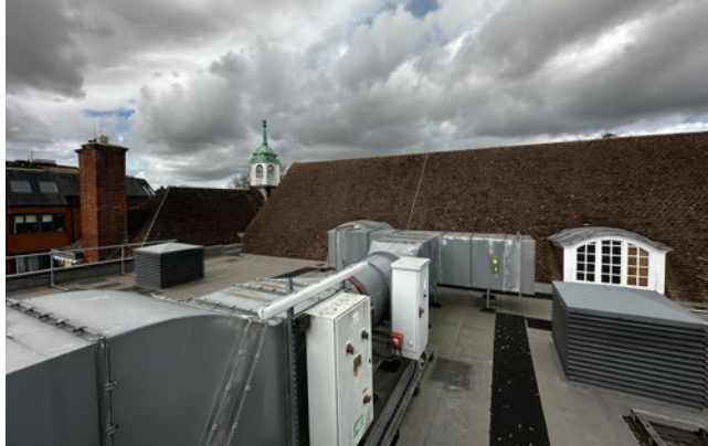
3.23 South end of Town Hall roof from museum extension flat roof
