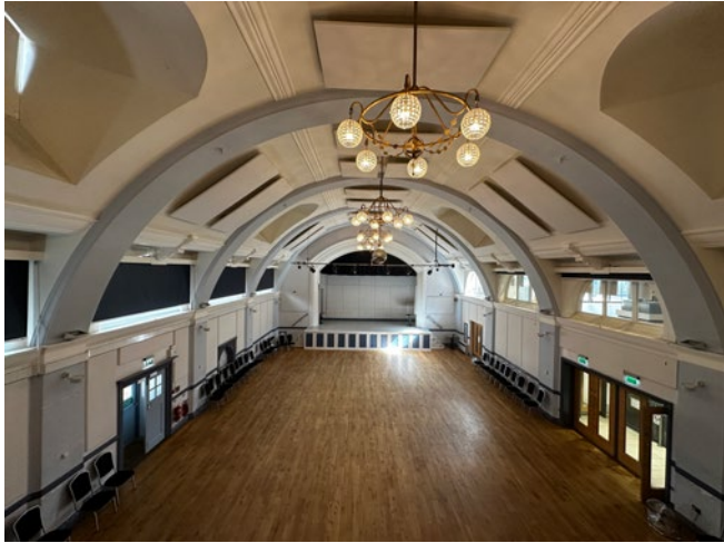
3.45 Looking north in G4 from balcony
