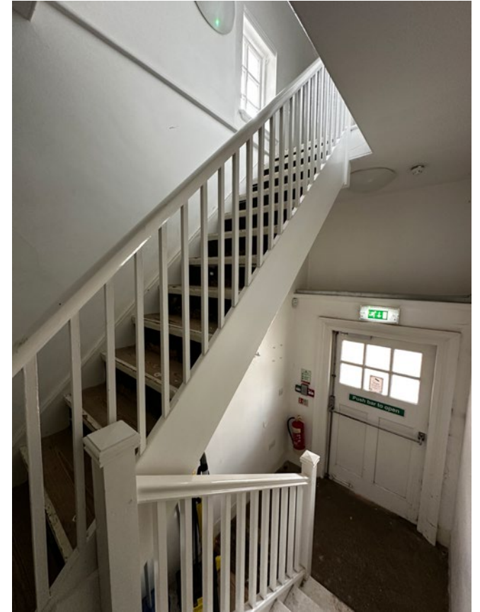
3.54 Looking west in G7 staircase
