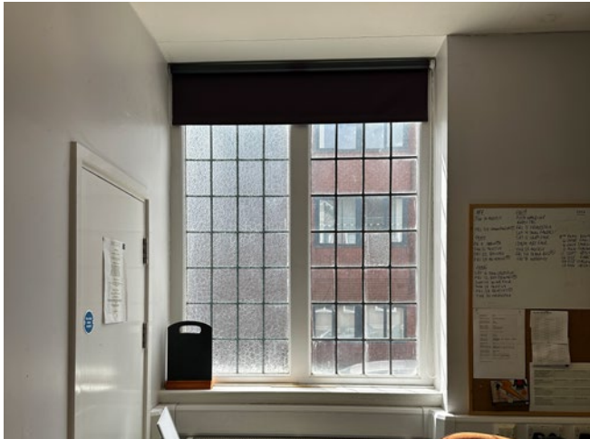
3.41 Detail of fixed casement leaded window in G2
