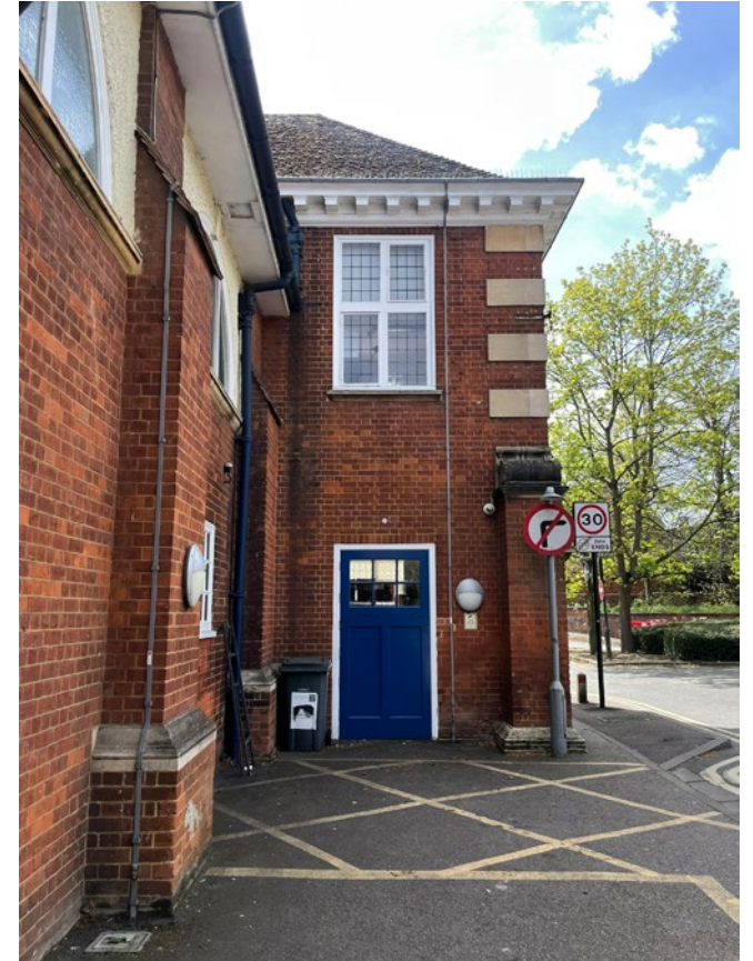
3.15 North elevation of projecting front range
