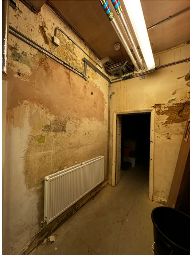
3.30 Looking south-west in B2
