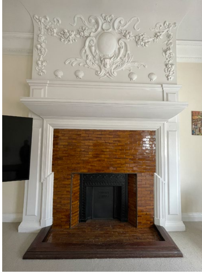
3.74 Detail of fireplace and overmantle in F4
