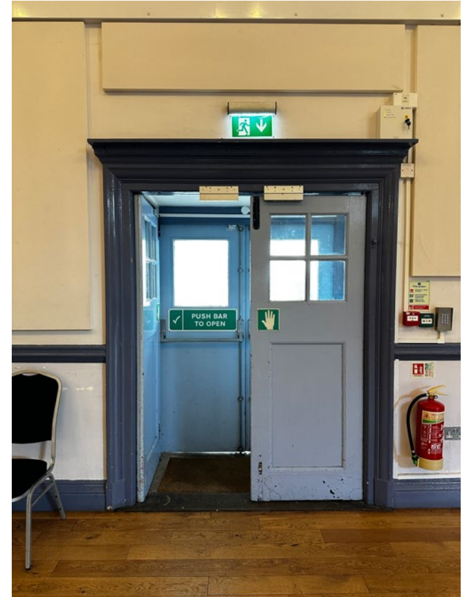
3.51 Detail of original double doors
