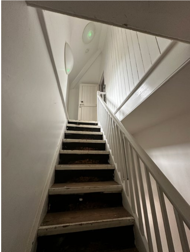
3.76 Stair to F5
