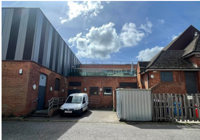
3.20 Looking at the central part of the north elevation
