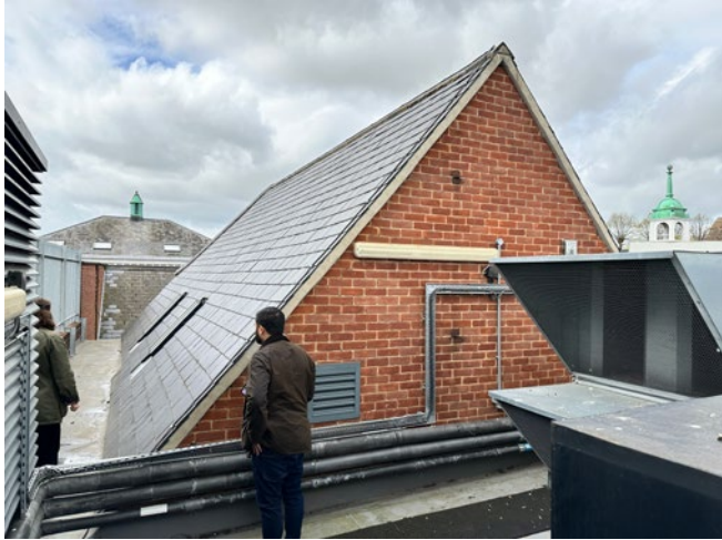
3.25 Looking south at the east pitch of the Workmen's Hall
