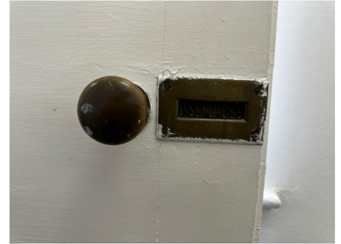
3.57 Detail of original door fittings
