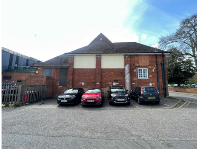
3.18 Looking at the west end of the north elevation (rear of stage)
