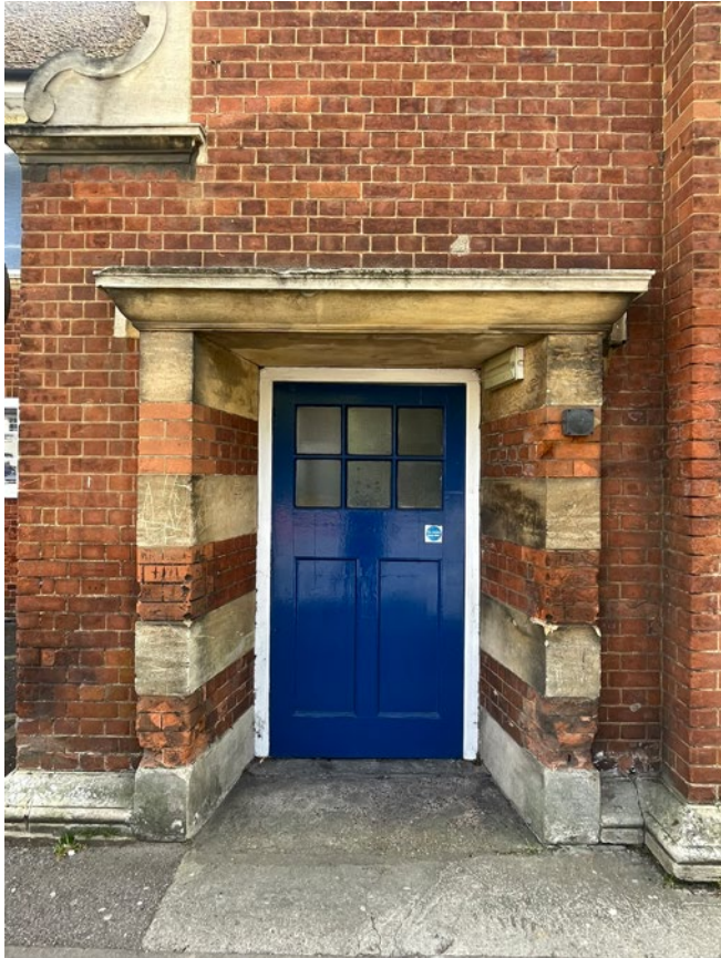
3.13 Door in west elevation to front range
