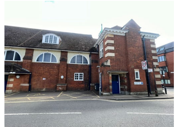
3.12 South end of west elevation
