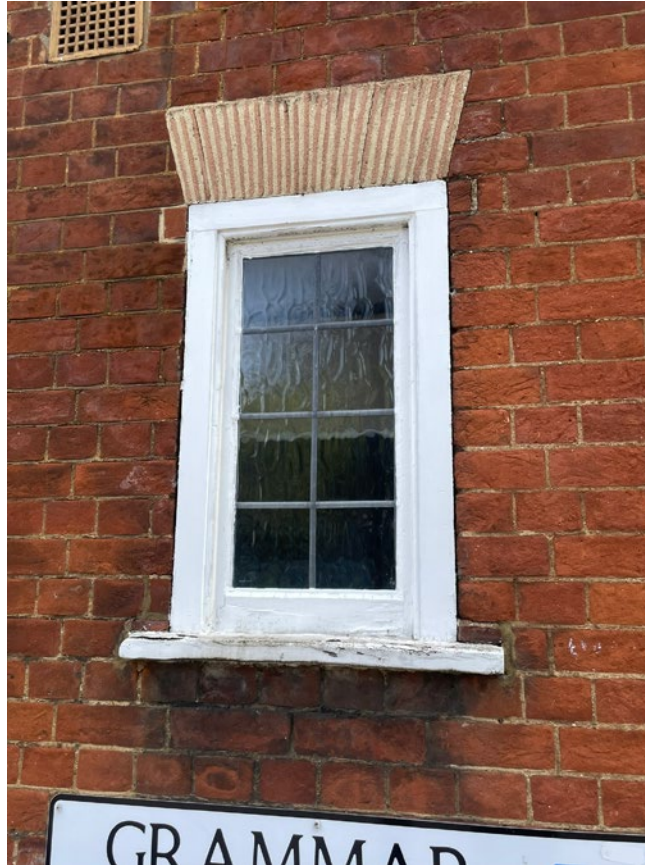
3.14 Detail of window in chimneystack of west elevation of front range
