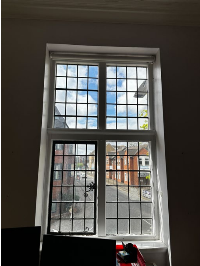
3.69 Detail of original 1900-1 window with latch and axial hinged toplight
