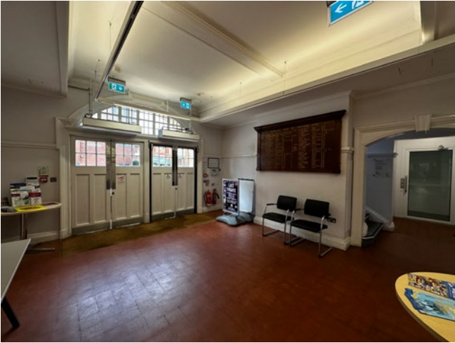
3.36 Looking south-west in G1
