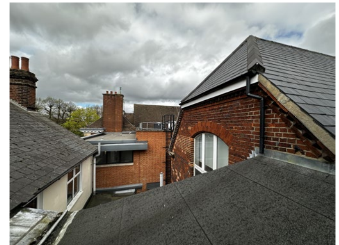
3.9 South elevation of the 1868 Workmen's Hall
