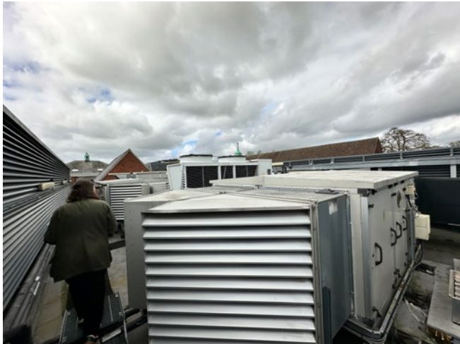
3.28 Looking south from the former gym flat roof to the Workmen's Hall
