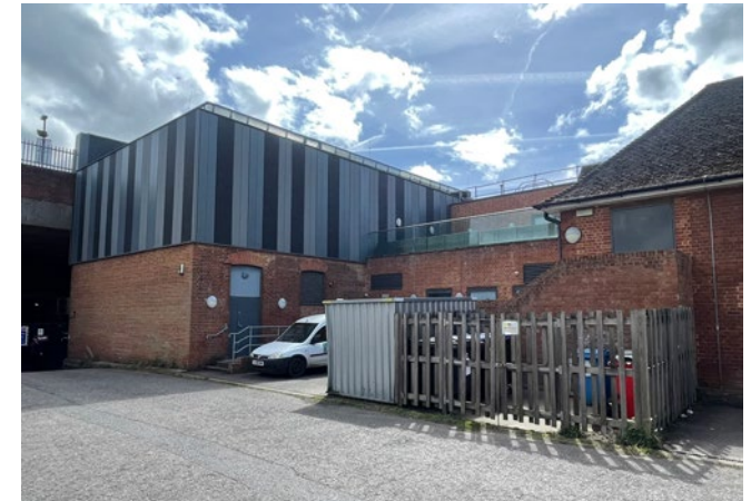
3.21 Looking at the east end of the north elevation, comprising the former early 20 th -century gym and modern first-floor museum extension
