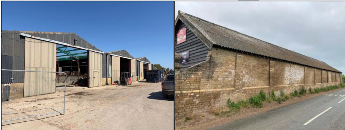
Figure 2 - L: Modern Barn. R: Gault Brick Barn
