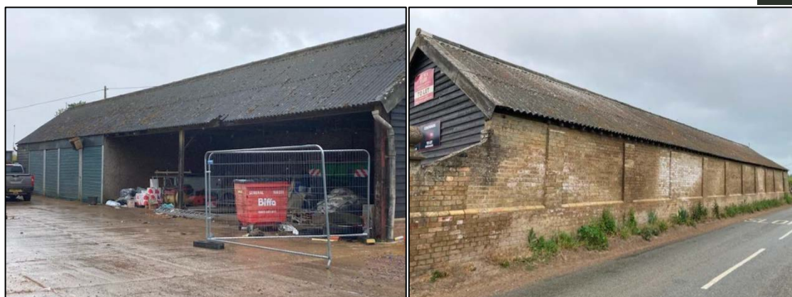
Figure 3 - Existing Gault Brick Barn
