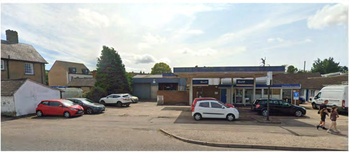
Existing Petrol Filling Station Street View
