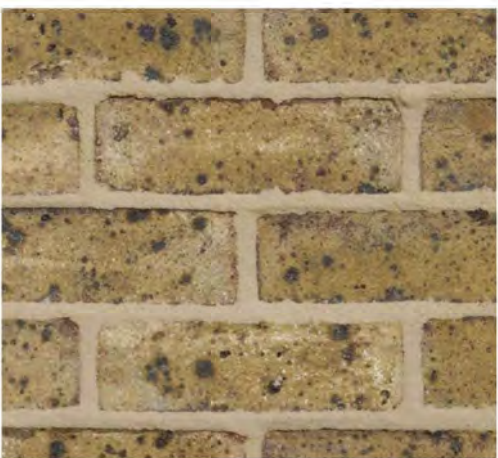
Facing Brickwork: stock brick (buff)
