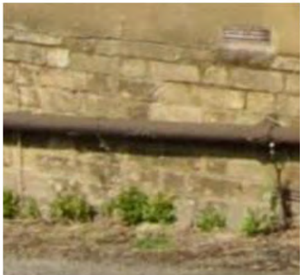
Facing Brickwork: (buff)
