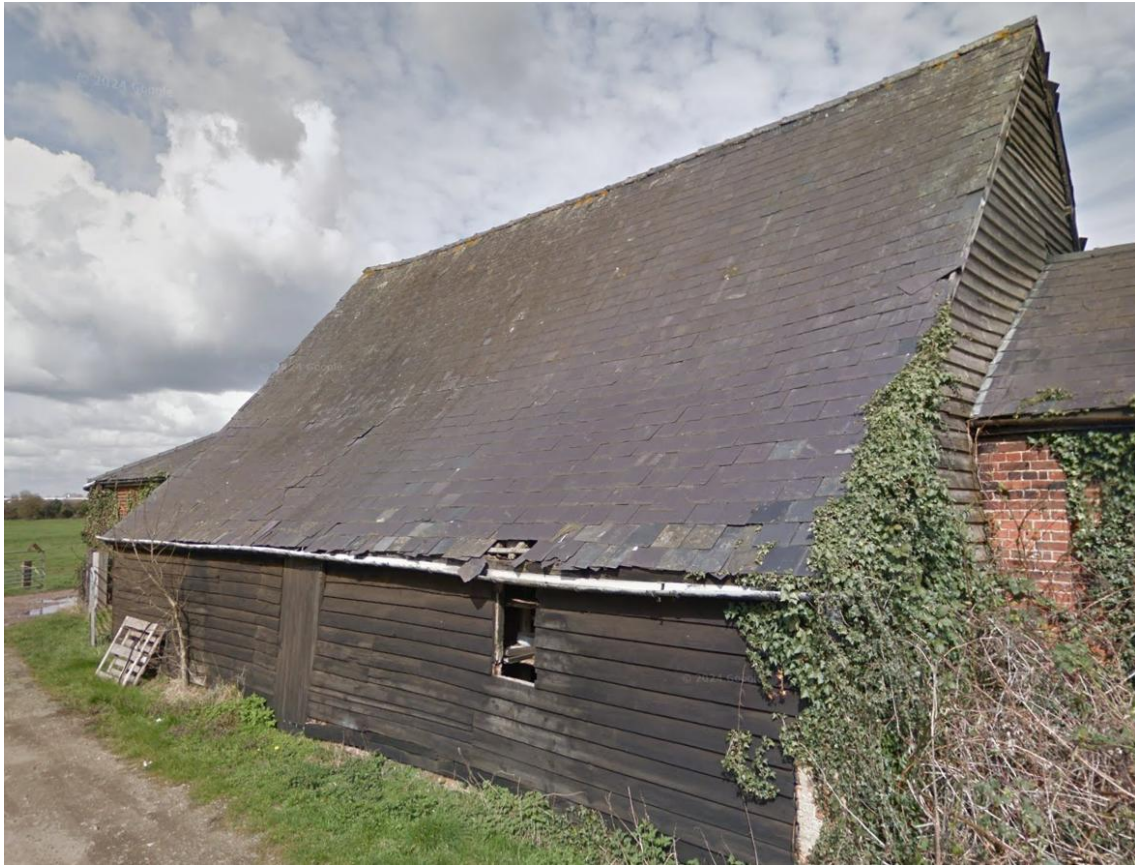
Figure 6 - Unit 2 Rear Roof Slope
