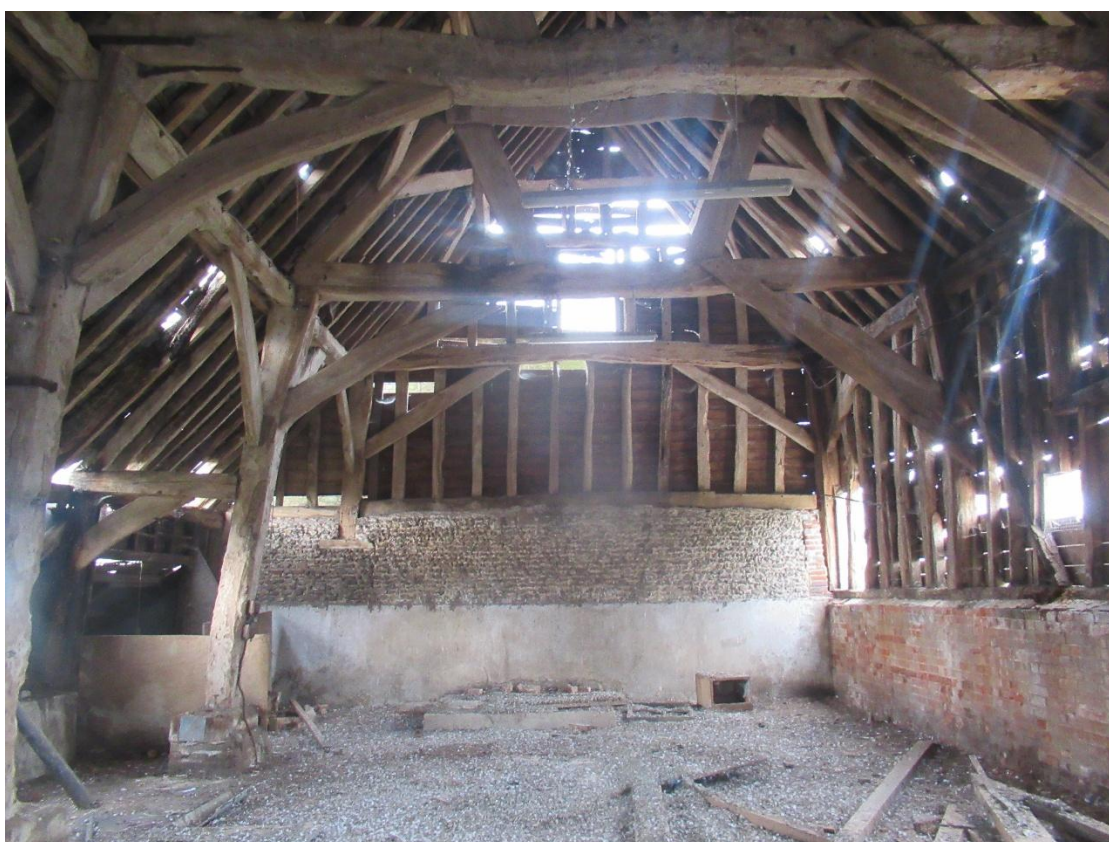
Figure 4 - Threshing Barn Internal
