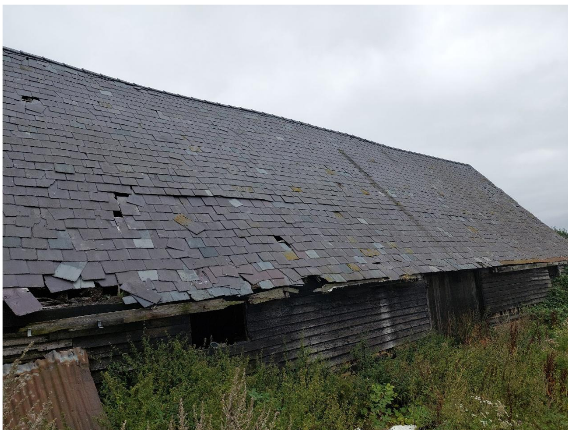
Figure 3 -Threshing Barn Rear Roof Slope
