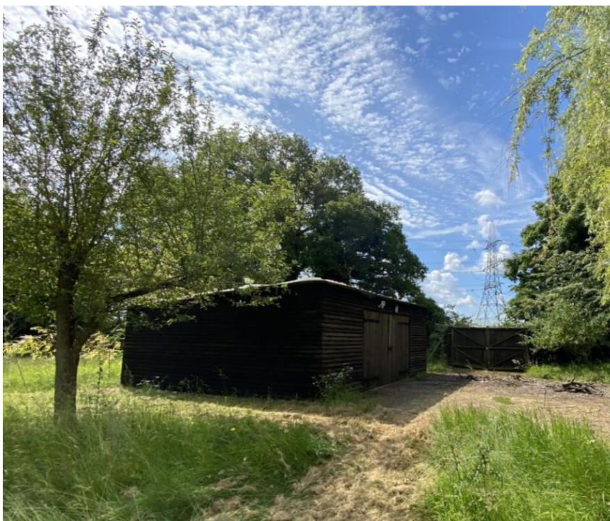
Figure 6: Photo of existing garage onsite, to be demolished and replaced, taken June 21 st , 2024
