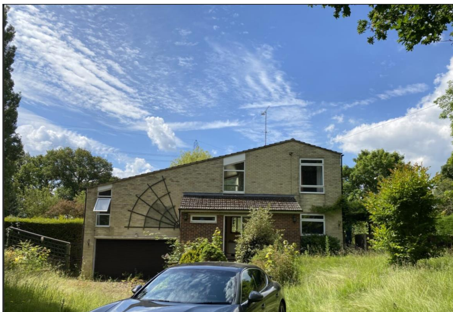
Figure 5: Photo of existing dwellinghouse, Ryefield, viewed from driveway off Stevenage Road, taken June 21 st , 2024
