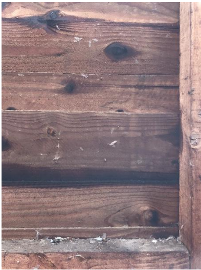
Plate 9: Wing casings along the interior walls of the garage
