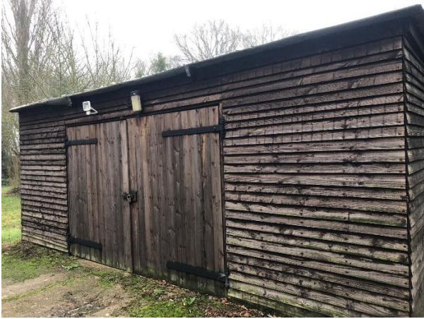
Plate 7: Existing garage (MR 3) showing security light and double doors with small gaps
