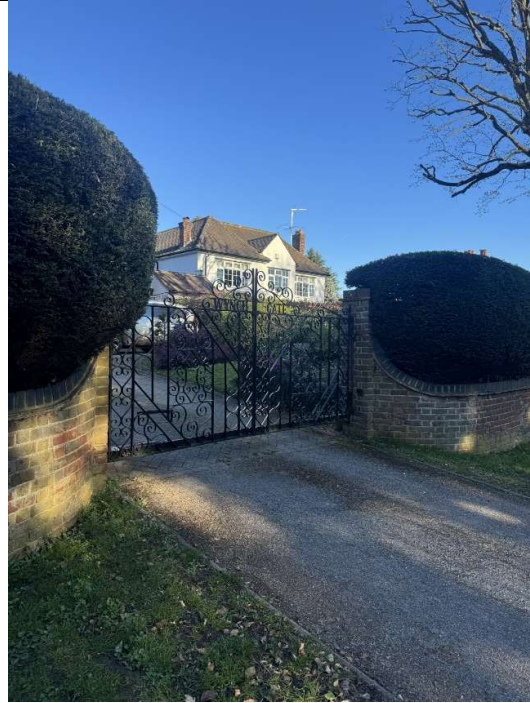
Photo 6: Brick piers exceeding 1.0m in height, together with a brick wall and setback black metal vehicular access gate.
