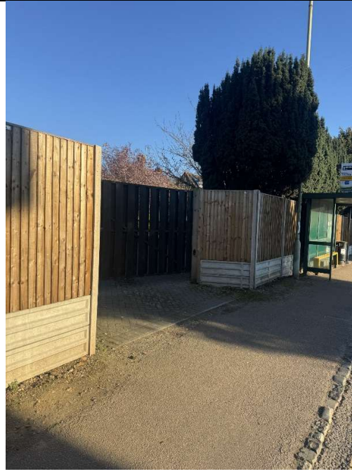
Photo 2: Boundary structure exceeding 1.0m in height positioned directly adjacent to footpath, including a vehicular access gate.
