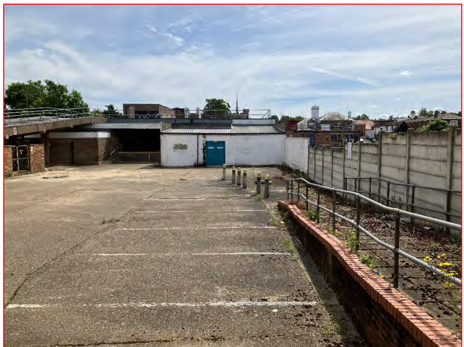
Plate 6: General view of ground floor car park and ramp to upper car park area (Dir. east)
