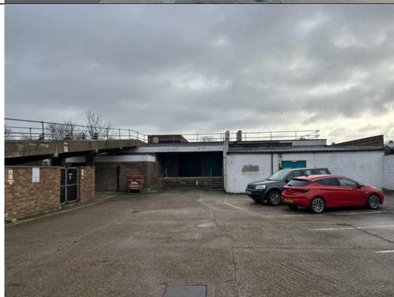
Photograph 3: Ground level car park located in the western side of the site
