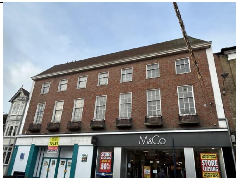
Photograph 1: Front of the building facing the high street
