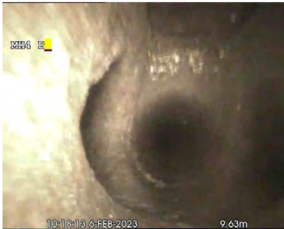
1aa8beed-8b10-4fb9-bd2a-54018b71e46a.jpg, 00:00:38, 9.83 m Junction at 3 o'clock, 100mm dia
