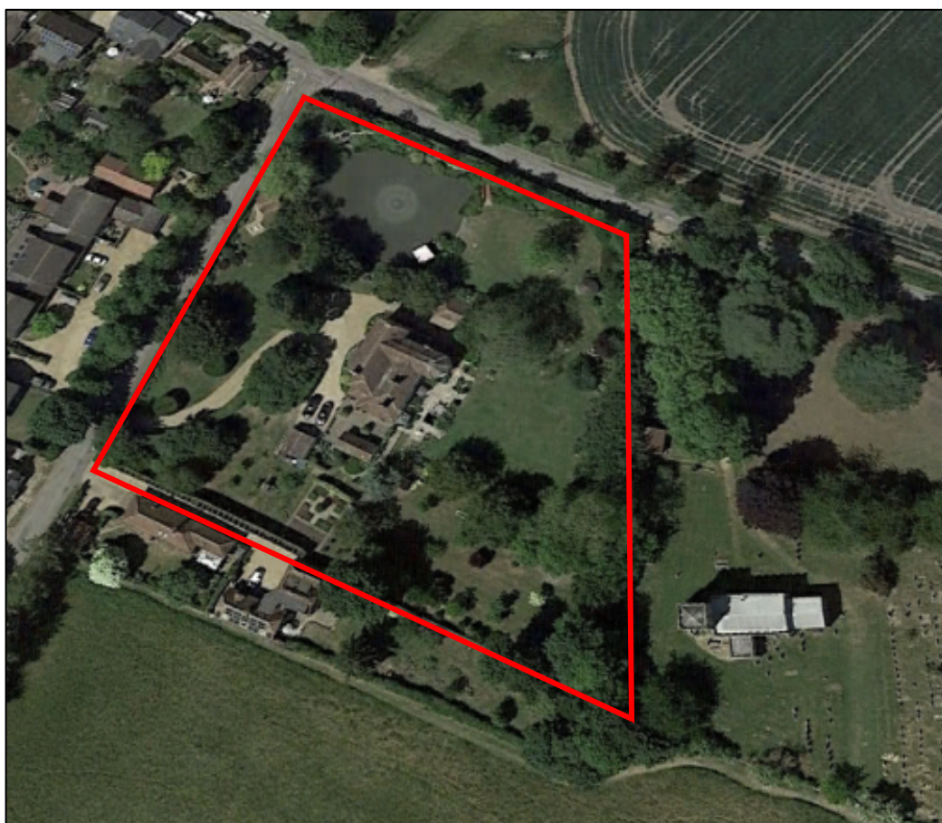
Figure 2 - The Application Site Close-Up
