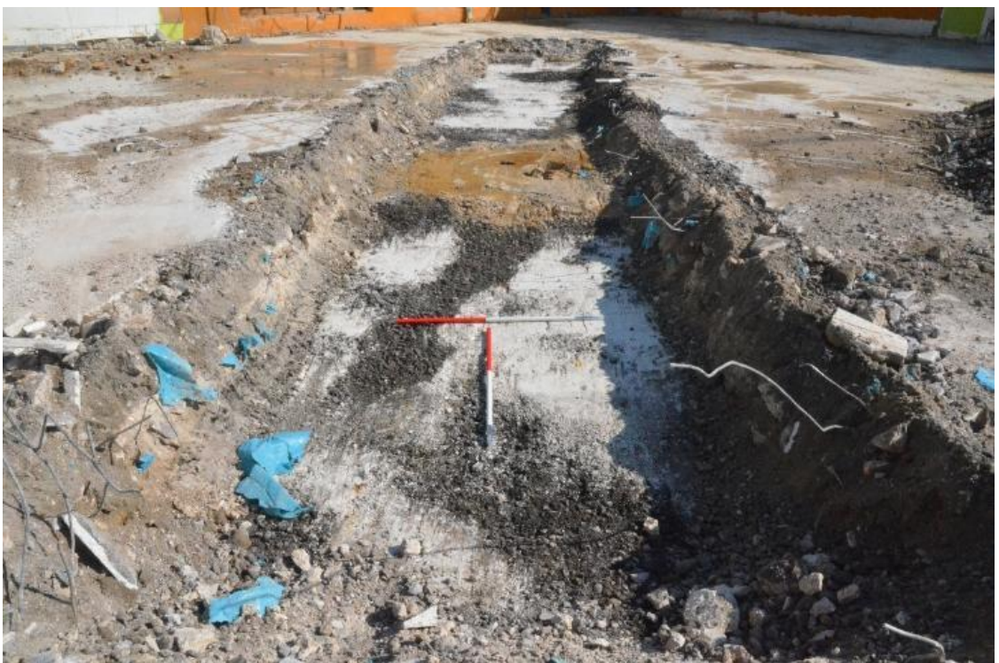
Plate 2: Trench 1, View Northeast
