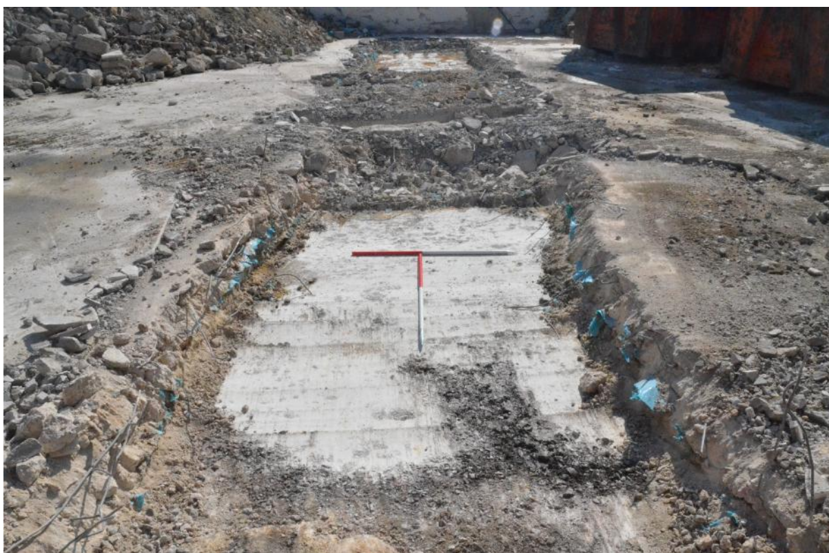
Plate 5: Trench 2; view South
