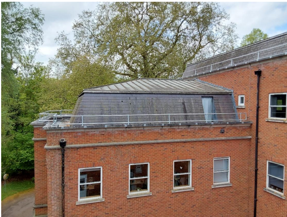
Photograph 2: South-east roof section
