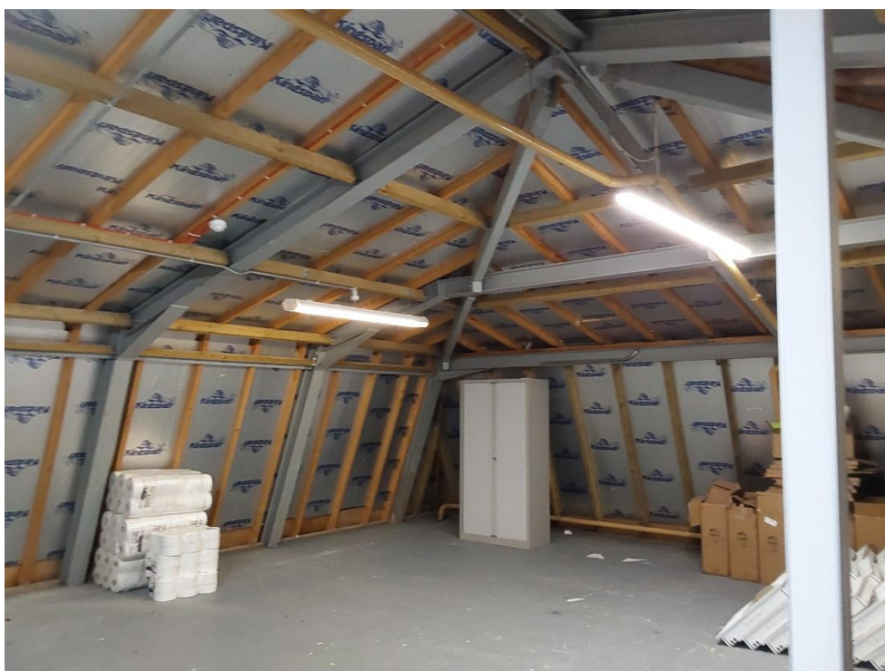
Photograph 5: Internal view of a roof cavity
