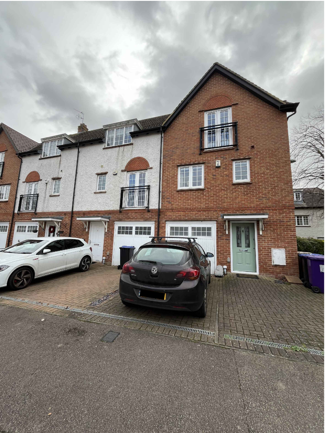
SITE PHOTO - FRONT ELEVATION
