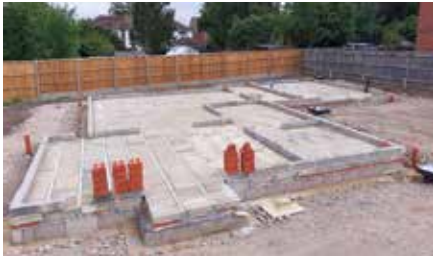
The foundations are prepared ready to receive the timber frame.
