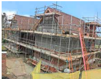
Followed by the external cladding.
