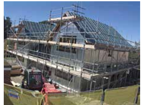
The roof is fully boarded, felted and counter battened by the shell erectors.
