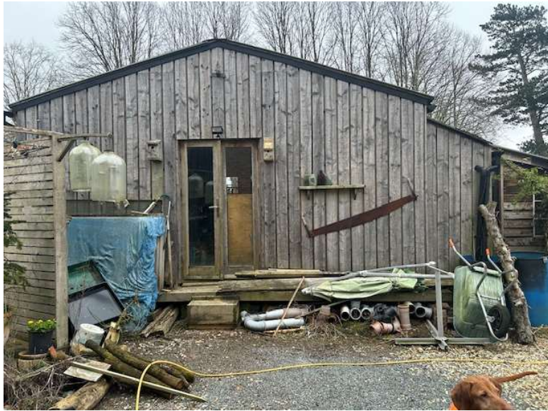
Photograph 1: Existing workshop to be demolished.
