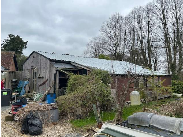
Photograph 3: Existing workshop to be demolished.
