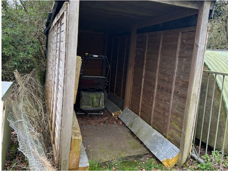
Photograph 7: Existing shed (2) to be demolished.
