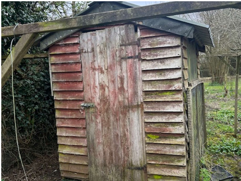
Photograph 8: Existing Shed (3) to be demolished.
