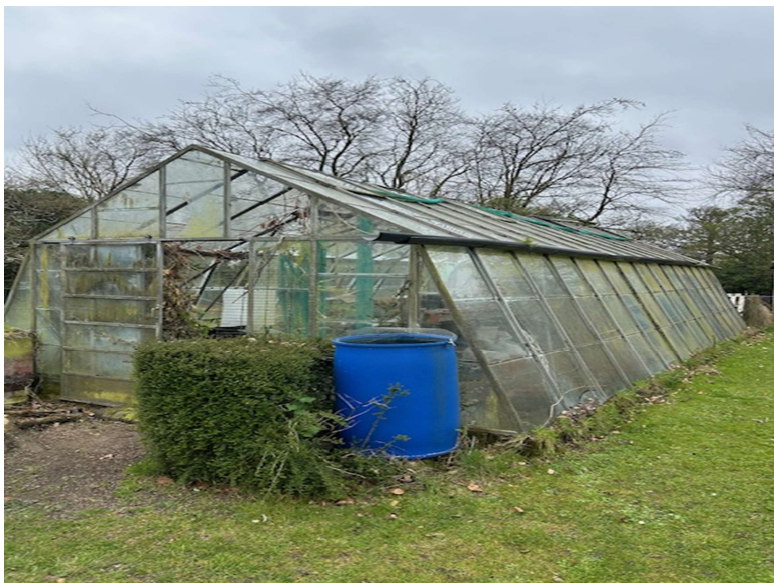
Photograph 4: Existing greenhouse (1) to be demolished.
