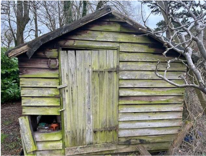
Photograph 9: Existing shed (4) to be demolished.
