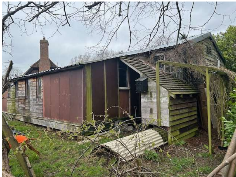
Photograph 2: Existing workshop to be demolished.
