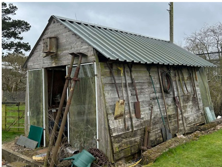
Photograph 10: Existing Shed (5) to be demolished.
