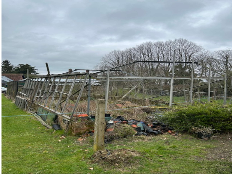
Photograph 5: Existing greenhouse (2) to be demolished.
