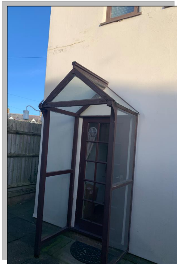
Photograph indicating the external door from the utility room to the south-west corner of the property. The outdated door joinery and porch can be seen, and relatively bland nature of the painted render walls.
