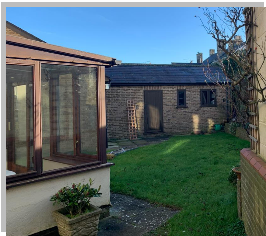
Photograph indicating the side elevation of the existing store facing the rear lawn and to the rear of the double garage to be converted into ancillary residential accommodation (guest bedroom/study).
