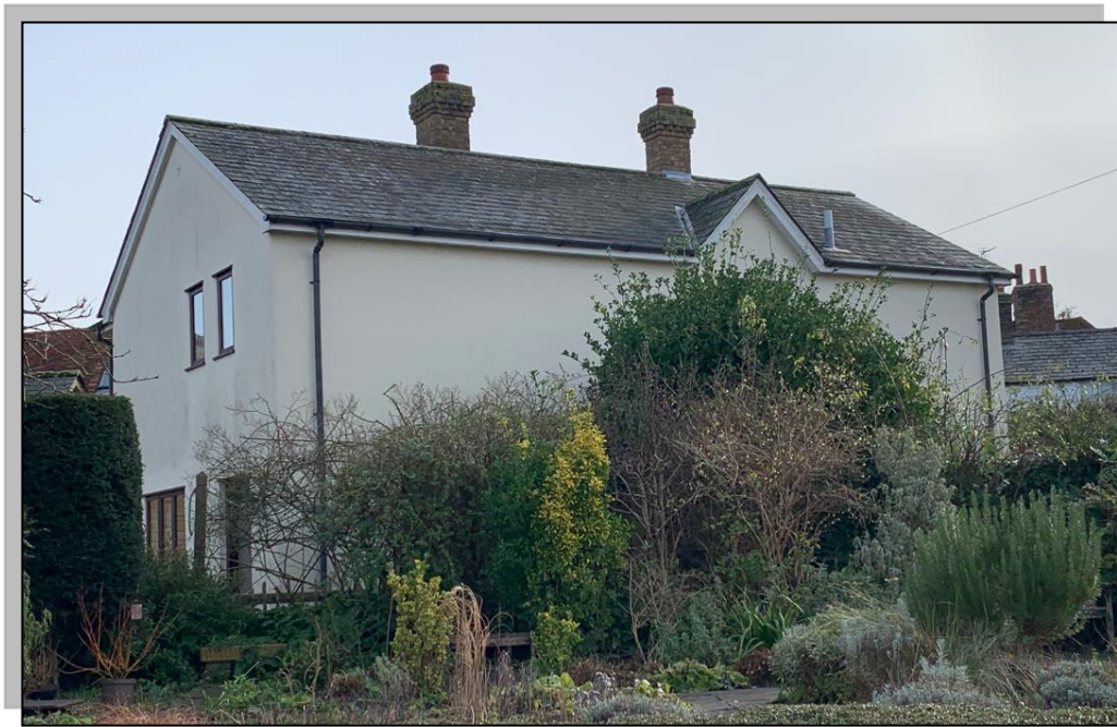
Photograph indicating the north-west elevation of the property.
