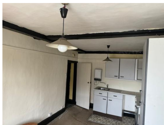
Internal views of 1 st floor bedroom & kitchen/lounge
