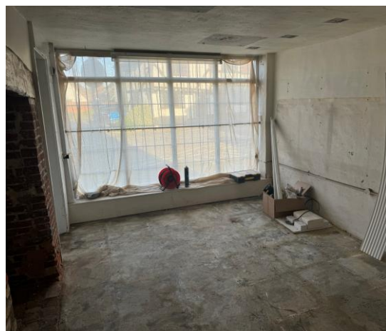
Views of ground floor interior – rooms to front
