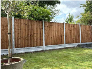
1.8m HIGH CLOSE BOARDED FENCE PANELS IN CONCRETE POSTS WITH CONCRETE GRAVEL BOARDS
