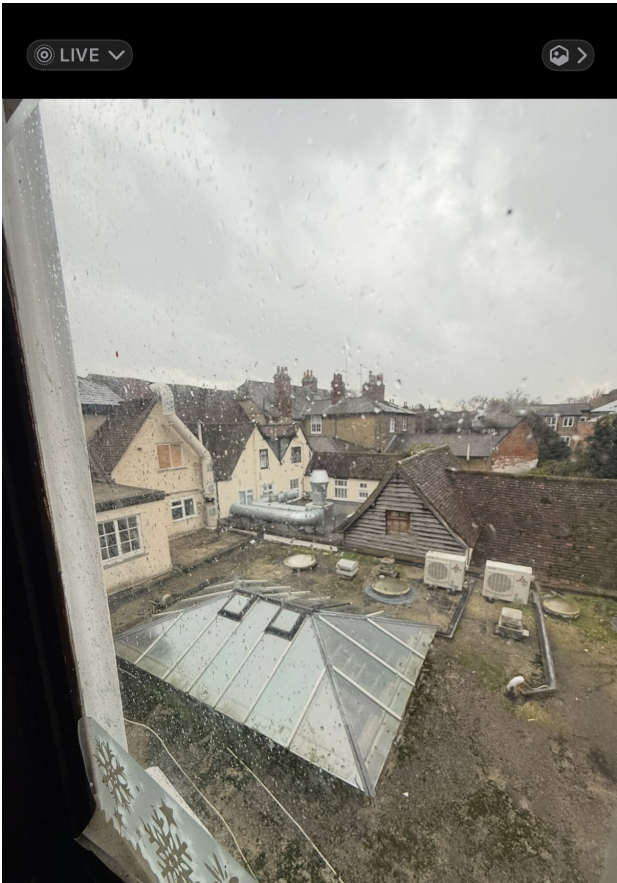
Fig. 8 — Wider context view of the backland area from 23 Market Place showing the concentration of roof-mounted plant, AC units and services across neighbouring commercial properties.
