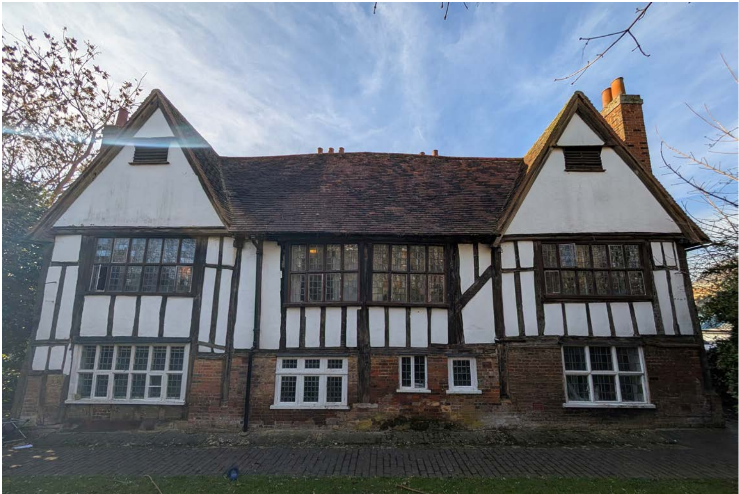
West elevation facing Queen Street
