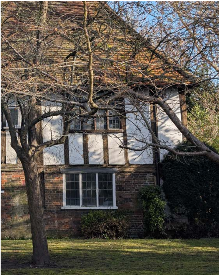
East elevation Viewed from the river
