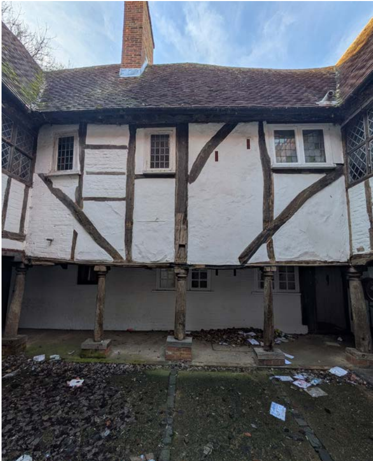
Internal Courtyard (east facing)
