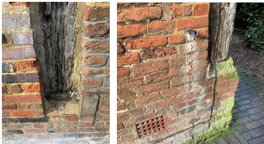
West and east corner posts of northern gable, eastern elevation
