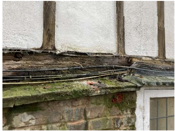
Saturated wall base along the western elevation, Downpipe discharge unknown, roofing felt flashings over first-floor plate, probable cement based render and impermeable paints
