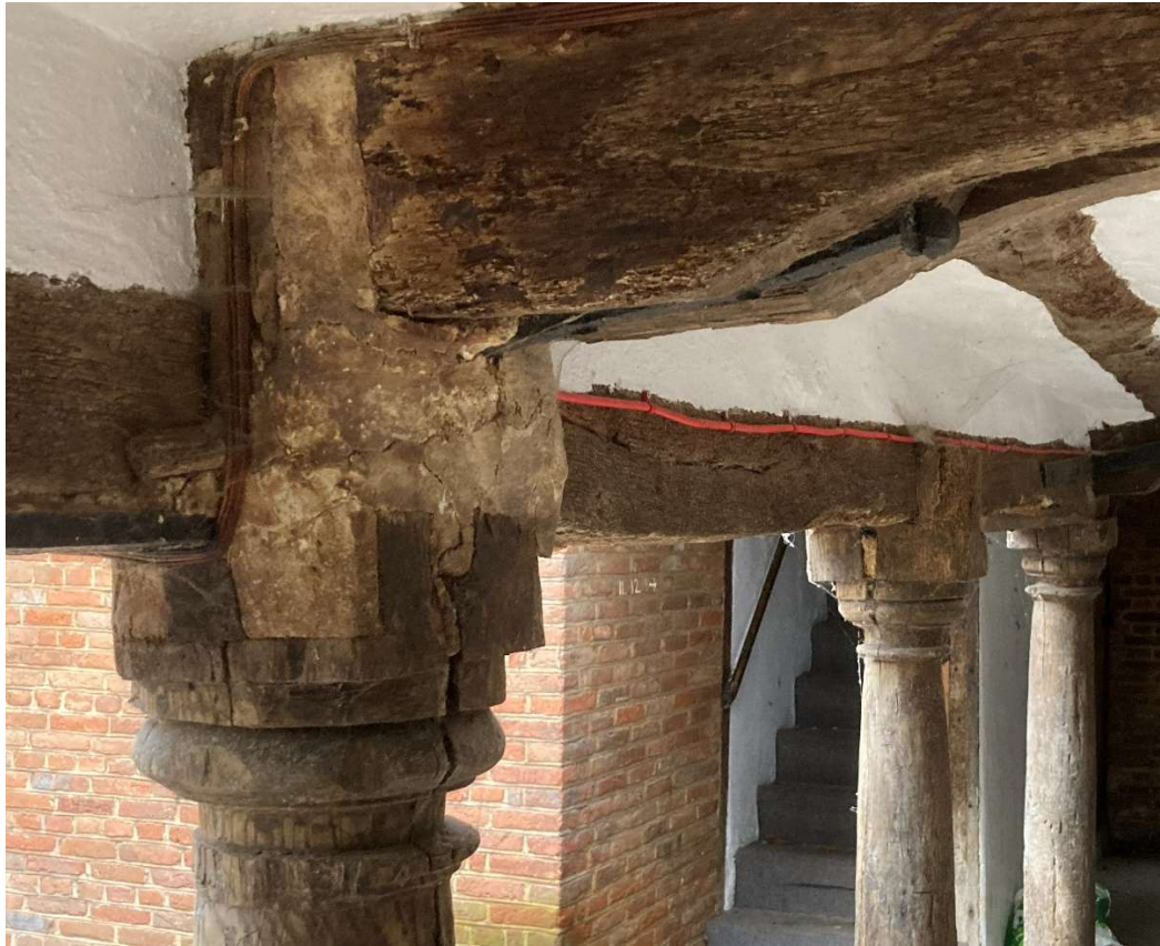
Timber filler to pack out the column heads
