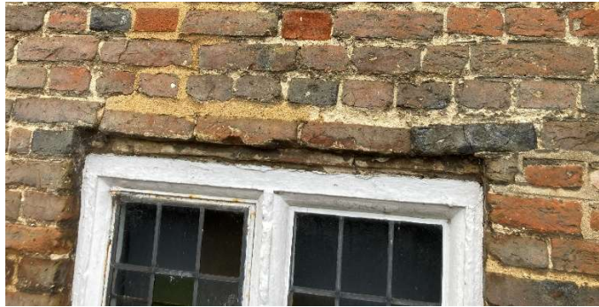
Continuation of stretcher course, dropped and supported by frame below
