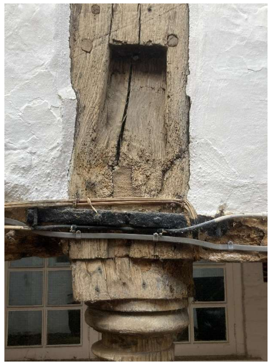
Pocket to provide means of temporary propping for repairs.
