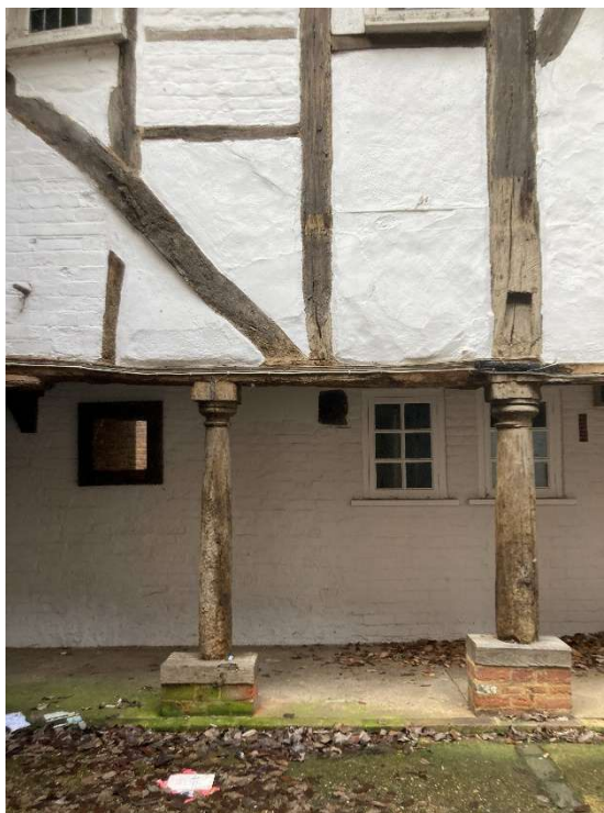
Pocket to provide means of temporary propping for repairs.
