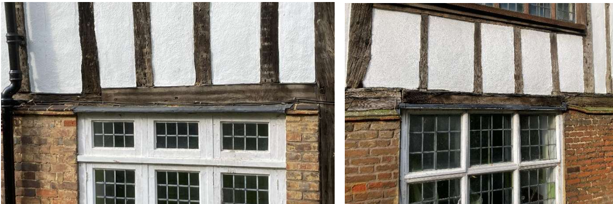
Oak repairs to the first floor plate stopping short of bearings
