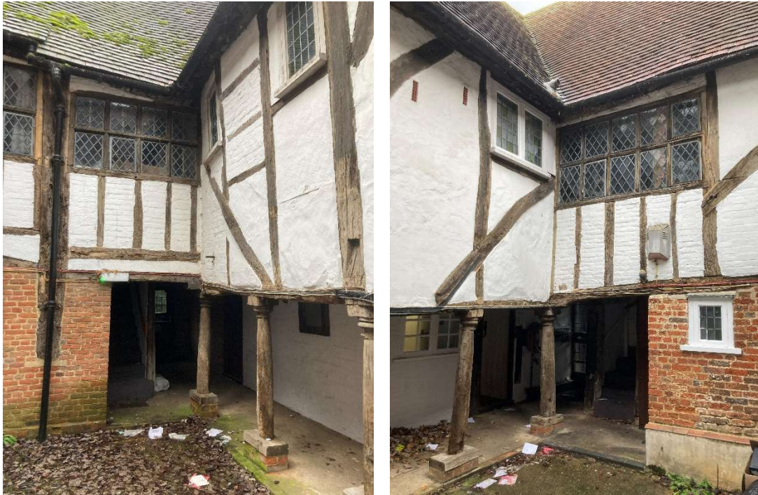
South and north sides of the cloister respectively
