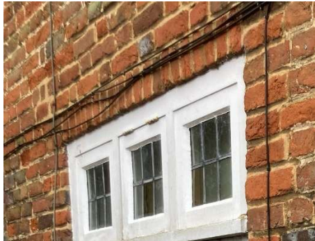
Rowlock course forming a flat arch lintol
