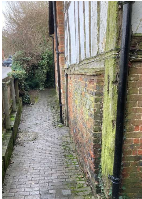
View along the face of the north elevation
