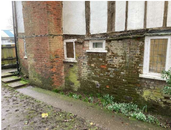
Saturated wall base along the western elevation, Downpipe discharge unknown, roofing felt flashings over first-floor plate, probable cement based render and impermeable paints
