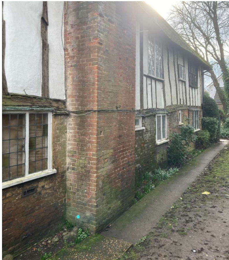
General view of west elevation, looking south
