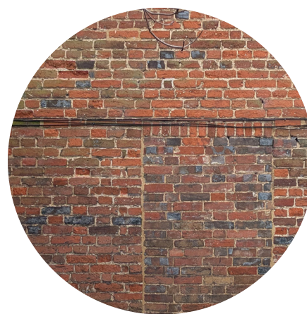
Brick Retaining Wall to match The Biggin in colour and texture
