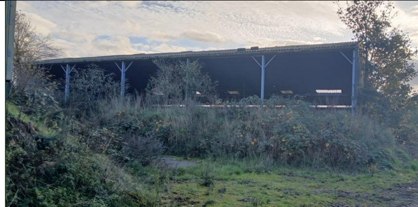
12 Open access of B2 along northern elevation
