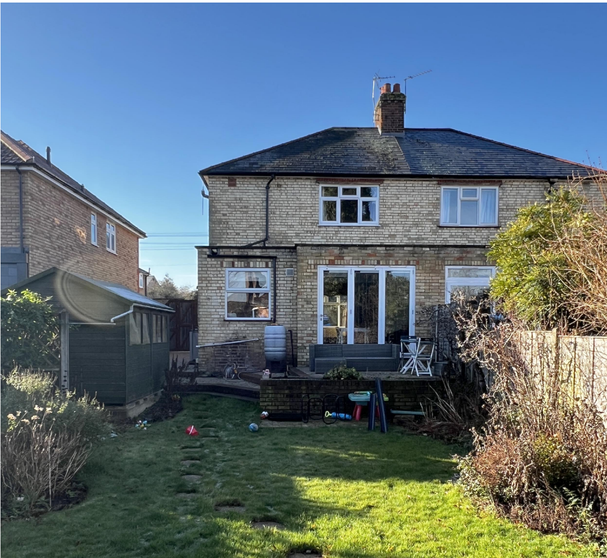
PHOTOGRAPH OF EXISTING REAR ELEVATION nts
