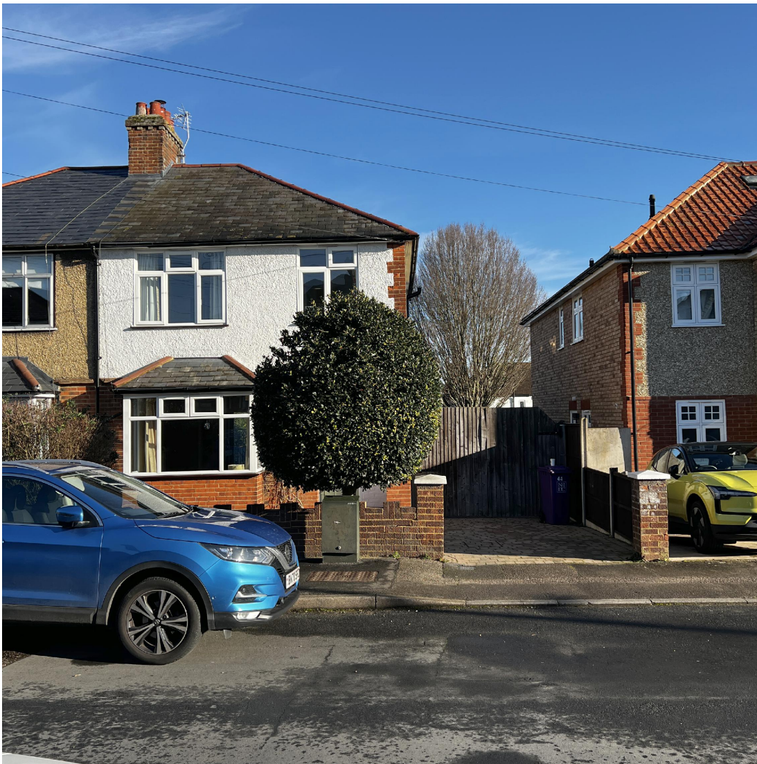
PHOTOGRAPH OF EXISTING FRONT ELEVATION nts
