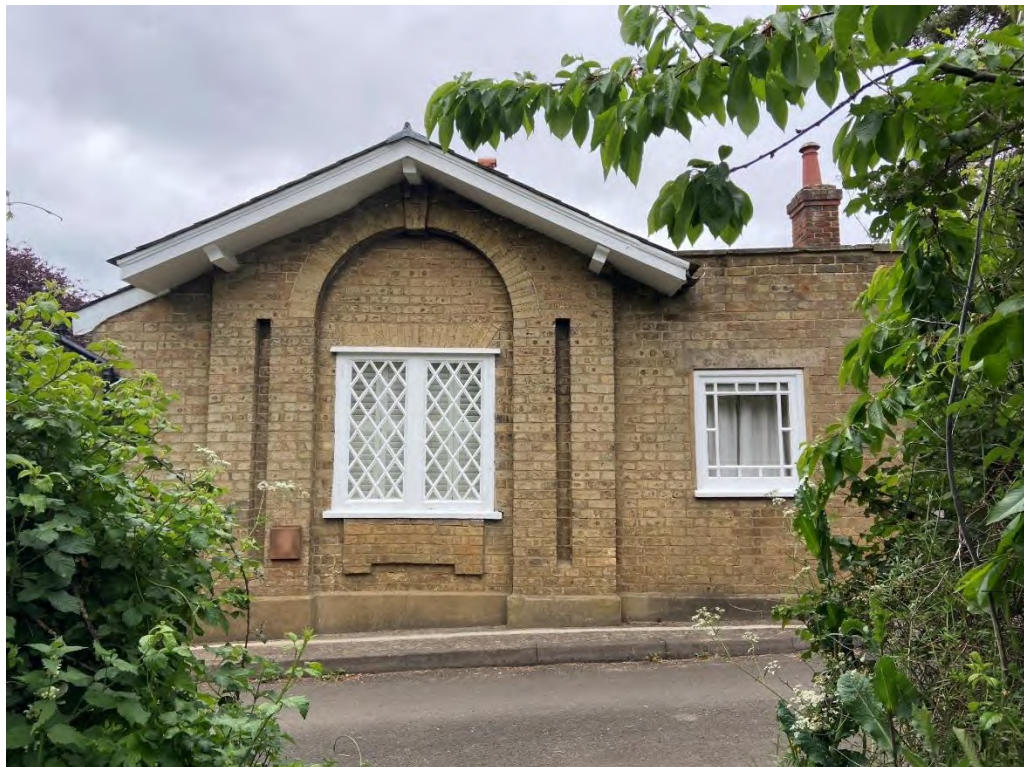
Photo 7: View of the south elevation of The Mill Farm, view to north-west
