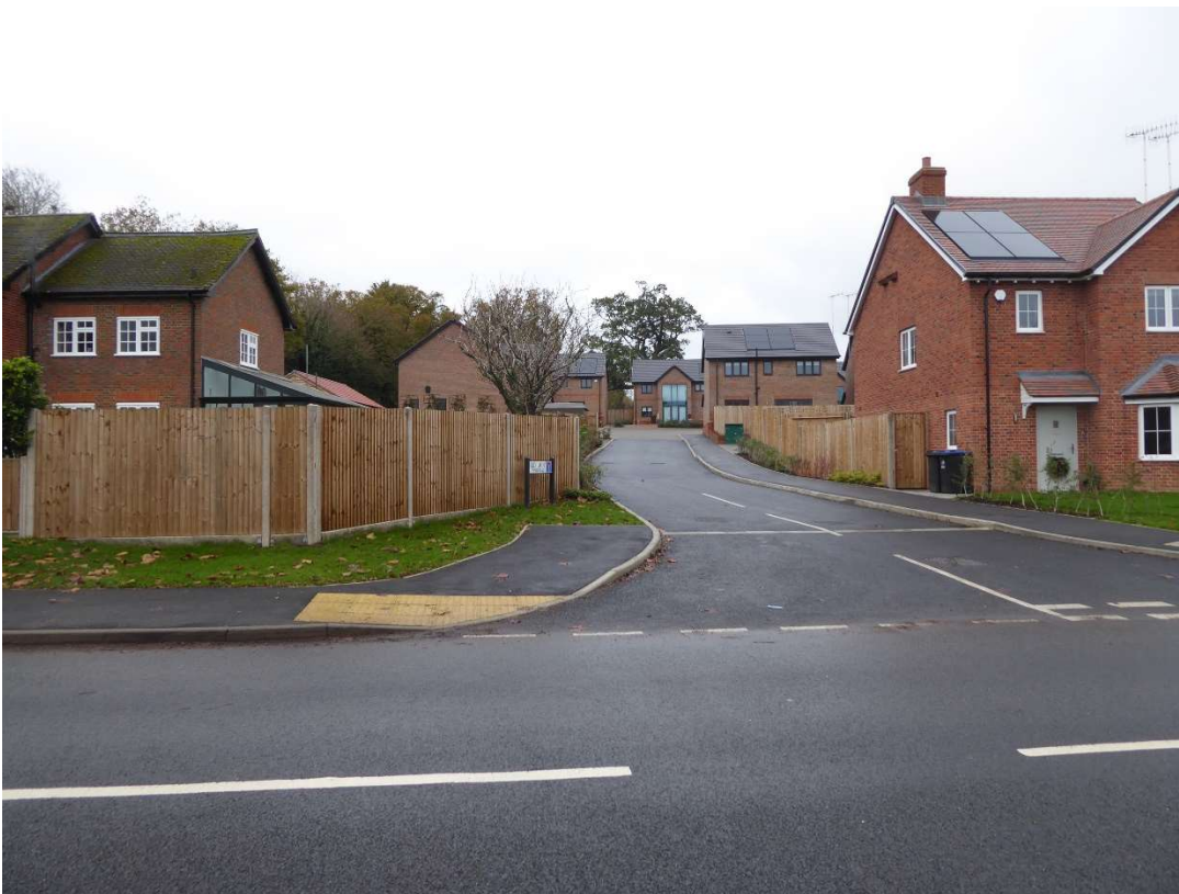
12. Entrance to the Jarvis Homes Development with pre-existing houses to the left
