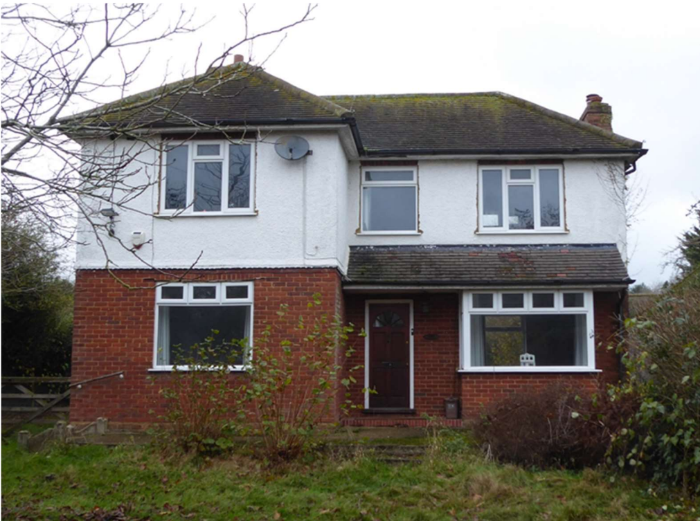
4. Front of the existing house
