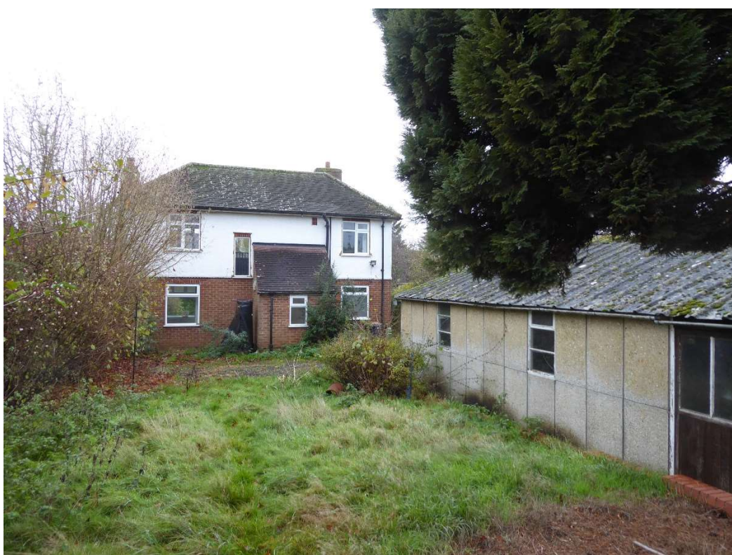
8. rear of the existing house and garage
