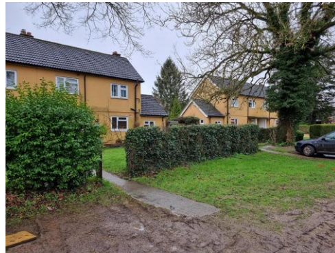
Semi-detached properties adjacent to site along Blacksmiths Lane with render and gables
