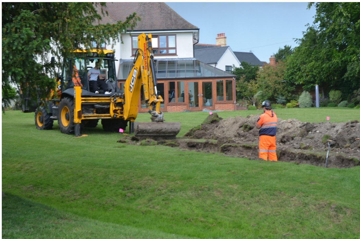
Plate 10. Machine excavation of Trench 3. View: Northwest.
