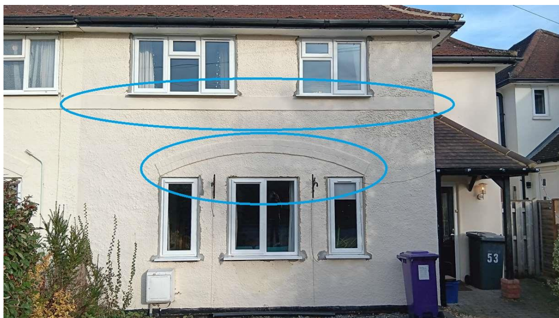
Front elevation existing decorative brickwork
