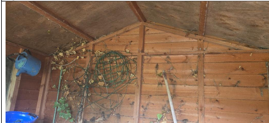
Figure 3: internal view of B2.
