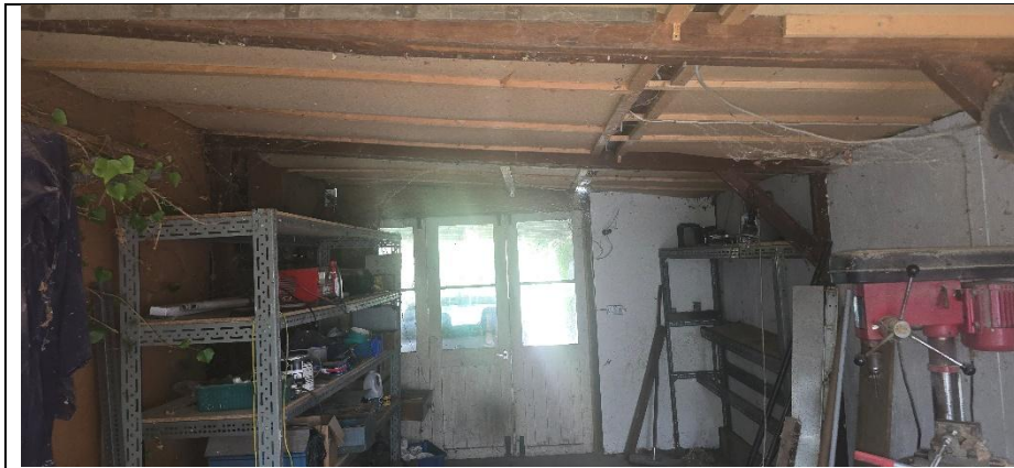
Figure 1: the internal look of B1.
