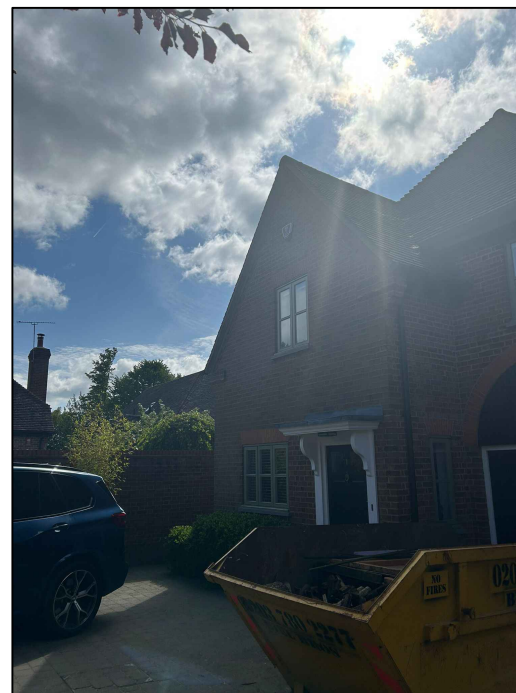
02 Site Photograph - Front Elevation
