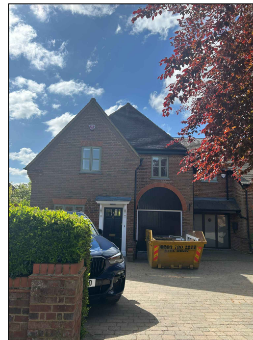
03 Site Photograph - Front Elevation
