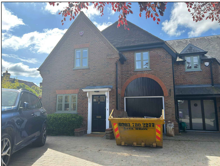
01 Site Photograph - Front Elevation
