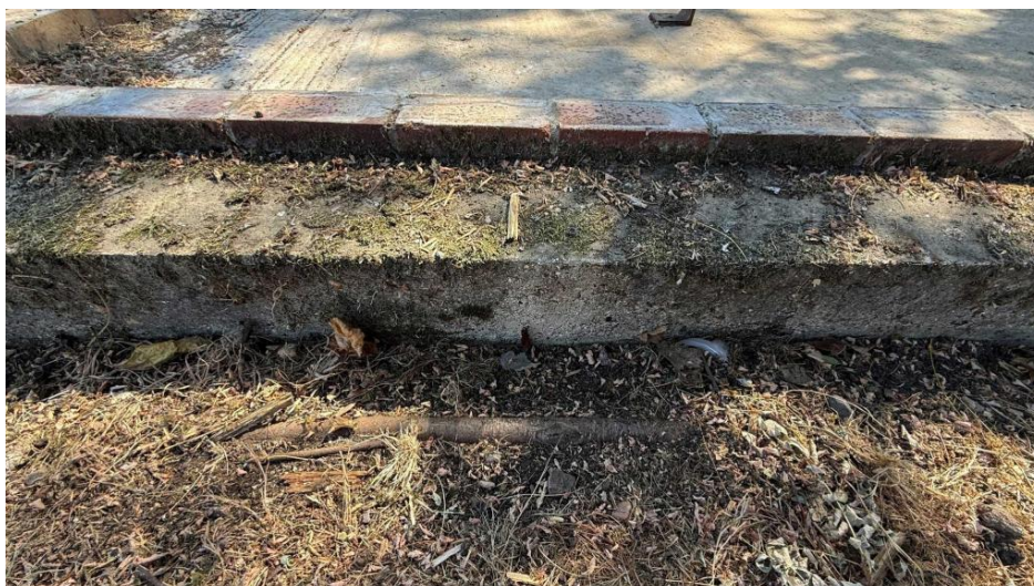
Roots and the edge of the old slab, illustrating the close physical relationship between R1 and the existing stable footprint.
