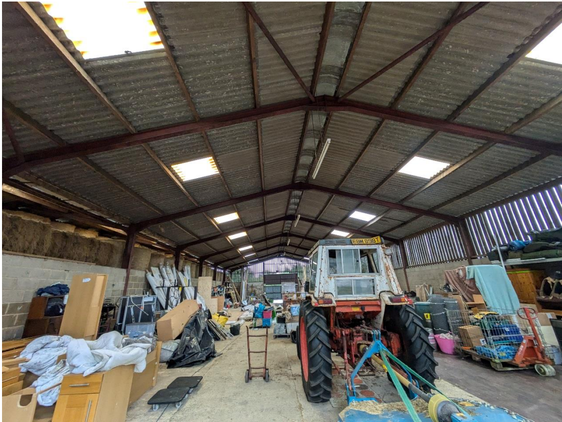
Photograph 3 Internal view of workshop/storage barn.
