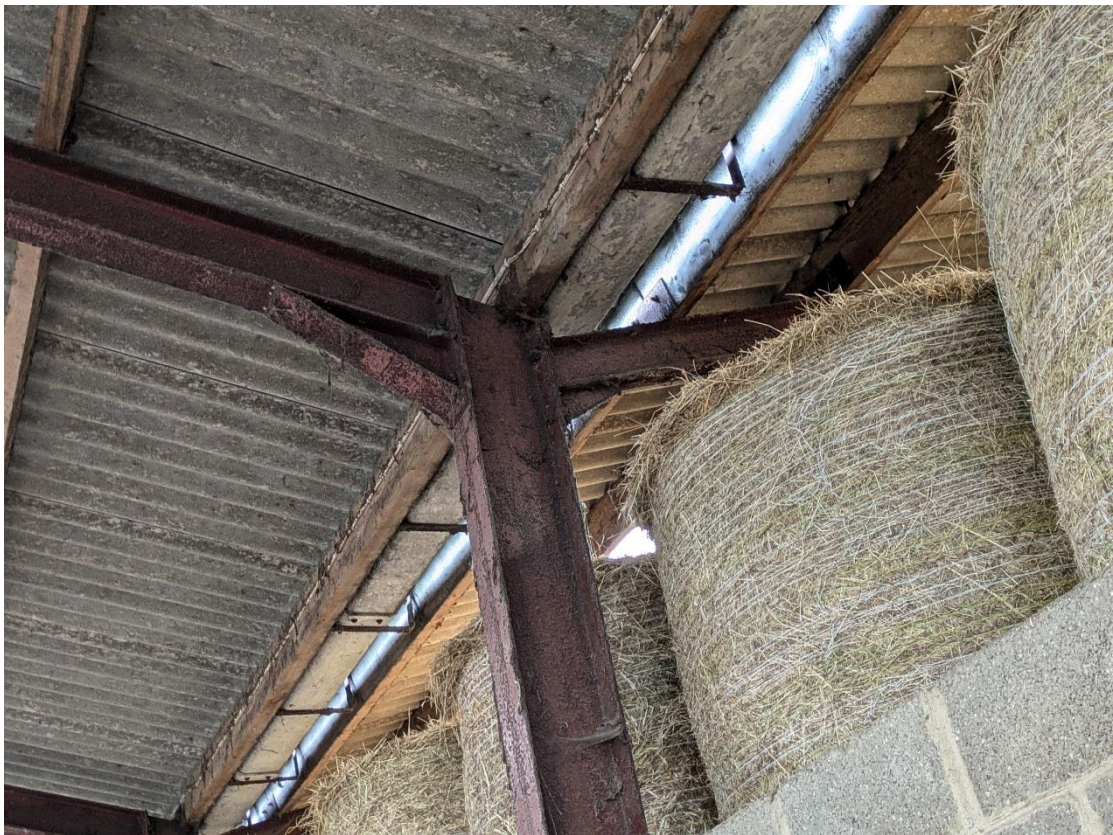
Photograph 4 Central post of double portal.
