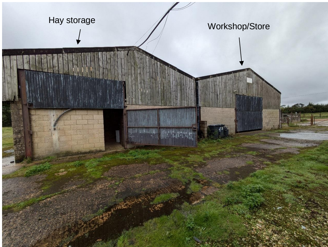
Photograph 1 View on front of barns.
