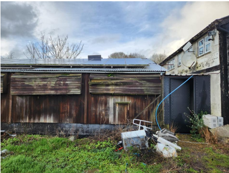
Plate B.2 Rear elevation of main farm building on-site (B1), showing timber cladding and potential roosting features.
