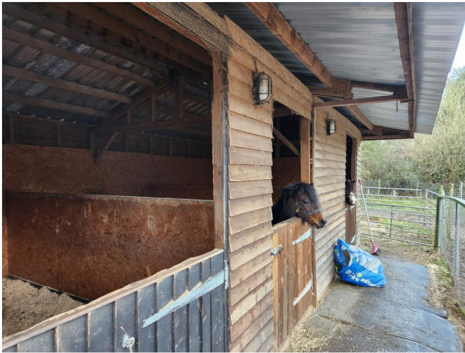
Plate B.9 Stables onsite, constructed of timber with open bays.
