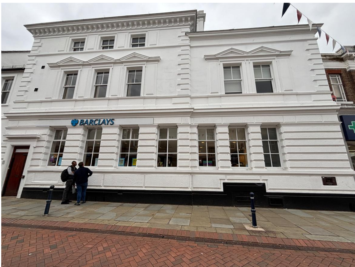
Existing Front Elevation Image
