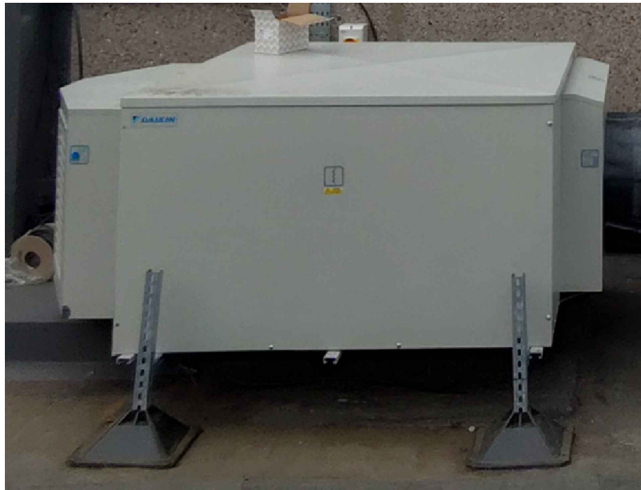
STOCK IMAGE OF A DAIKIN VAM2000FC EXTERNAL HEAT RECOVERY UNIT ON BIG FOOT STAND, WITHIN AN ADDITIONAL WEATHERPROOF HOUSING.
