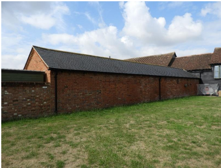
The blank brick wall of the rear wing to Rudwick Hall Barn along the application site boundary
