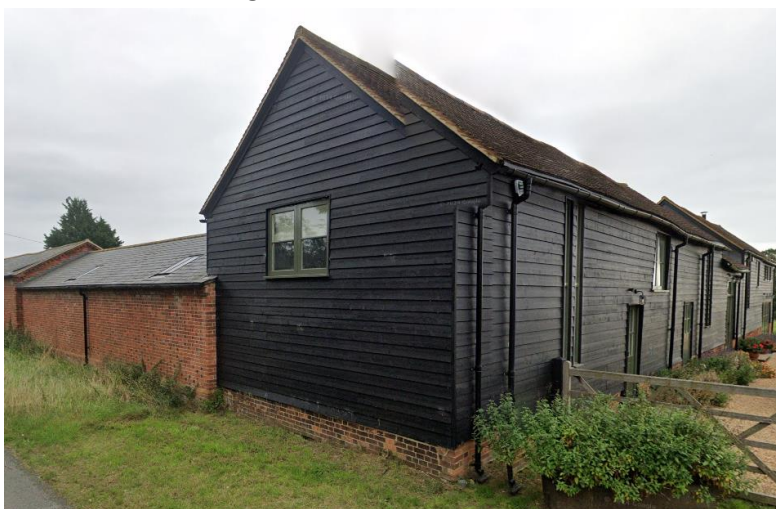
Oakley Barn: timber clad north-south range with brick wing to the east.
