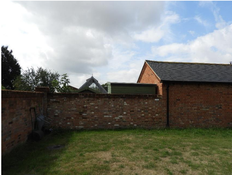
View across side boundary wall between Rudwick Hall Barn and Oakley Barn of storage shed and greenhouse within the garden of the former.
