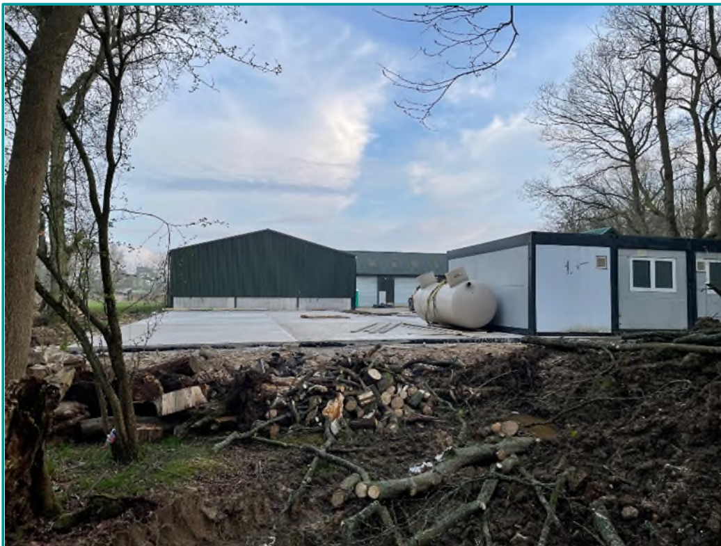
Figure 9: Showing tree removals
