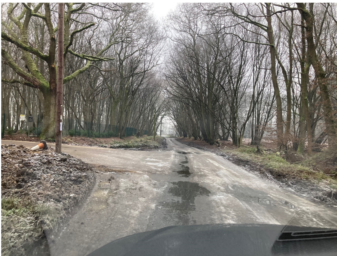
Photo 1: Three Houses Lane with site access drive on left, 12 January 2025
