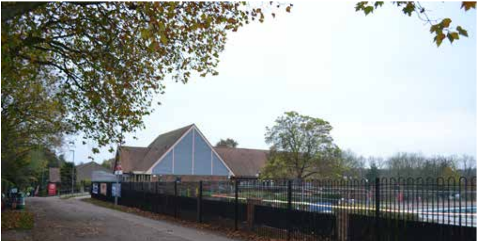
Figure 19 - View of the site looking south-west from the conservation area's eastern boundary on Elmside Walk.
