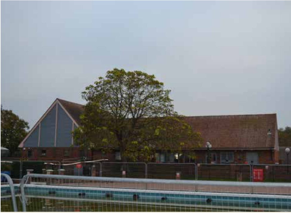
Figure 9 - View of the building from the locally listed swimming pool to the north.
