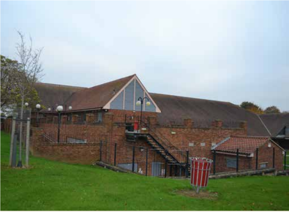
Figure 8 - View of the building from the north-west.
