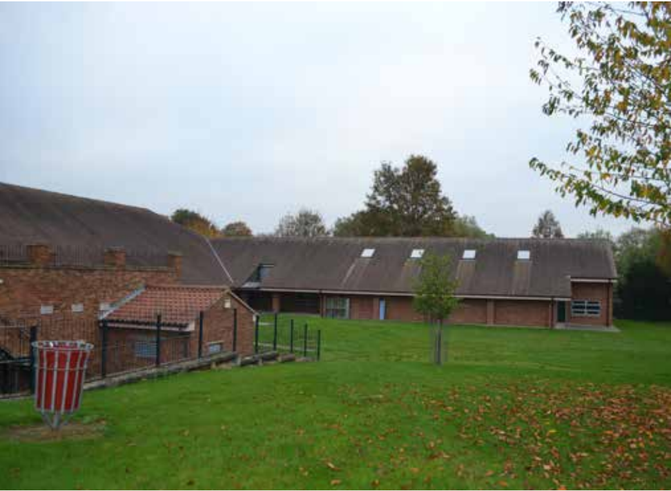
Figure 10 - View of the rear wing of the building from the north.
