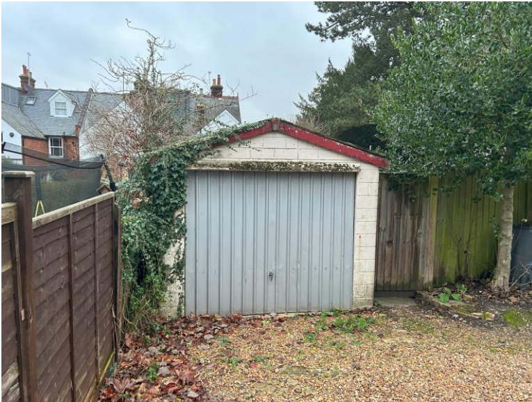
View of the garage store and parking area
