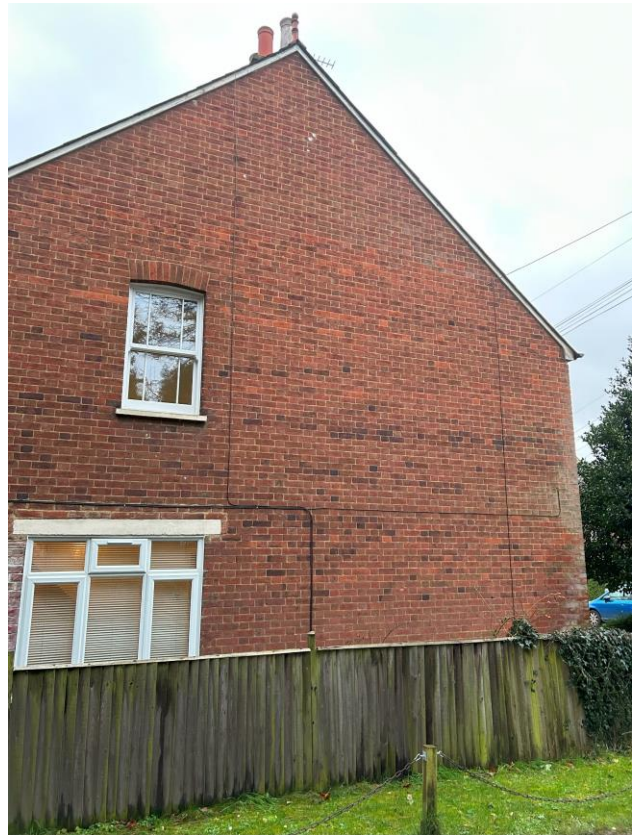
Closer view of the front of the side elevation showing the Upvc window to the dining room and timber sash to the bedroom above
