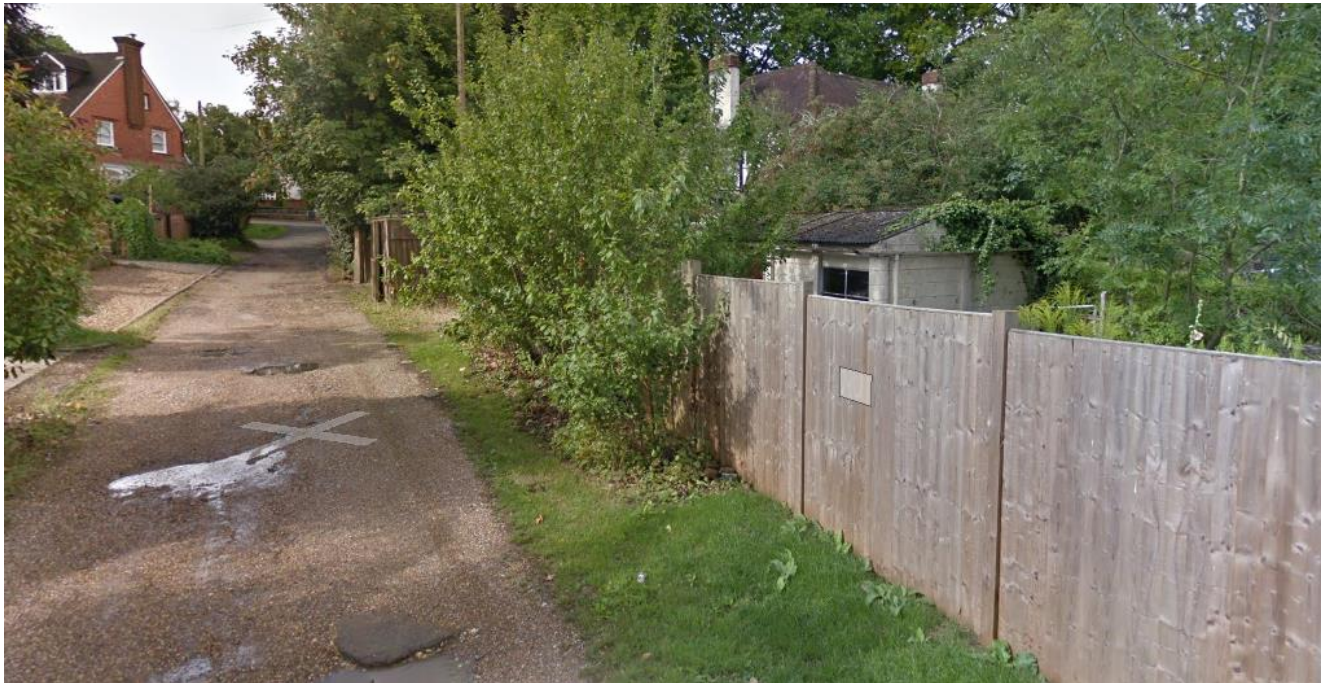
View along the side driveway showing the rear section of the garden fence and the garage store
