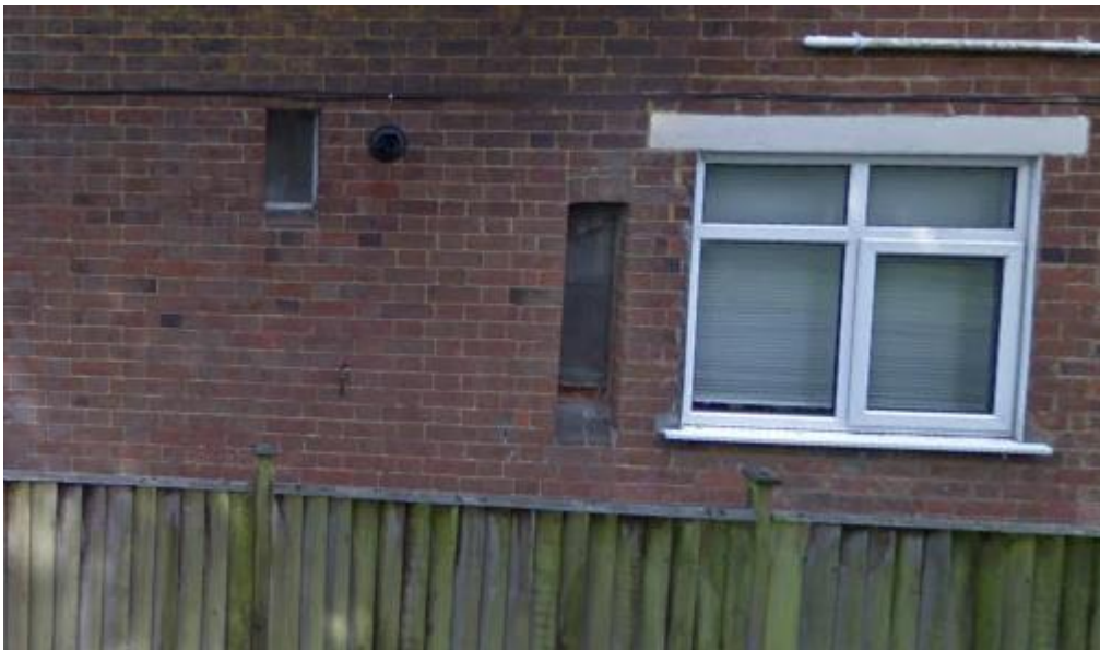
Photograph of the side ground floor kitchen window. This casement unit is in Upvc. To the left are the two narrow windows proposed to be bricked up
