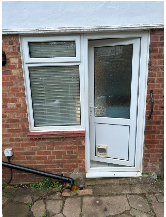
Close view of the ground floor rear Upvc external door and window
