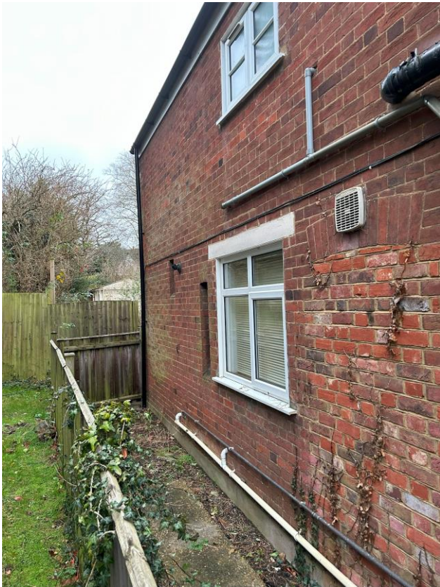
Closer view of the rear of the side elevation showing the Upvc windows to the kitchen and bathroom
