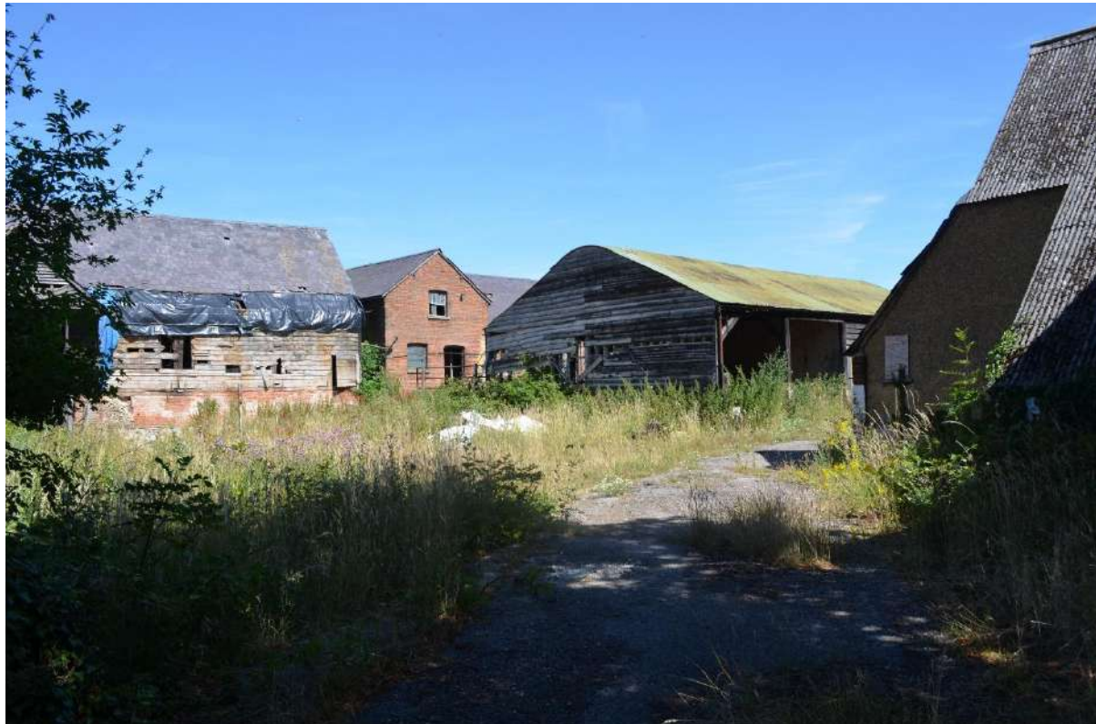
Plate 8: Farmyard courtyard buildings, view north.
