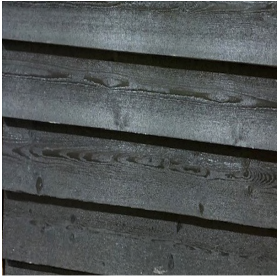
Timber weatherboarding (painted black)
