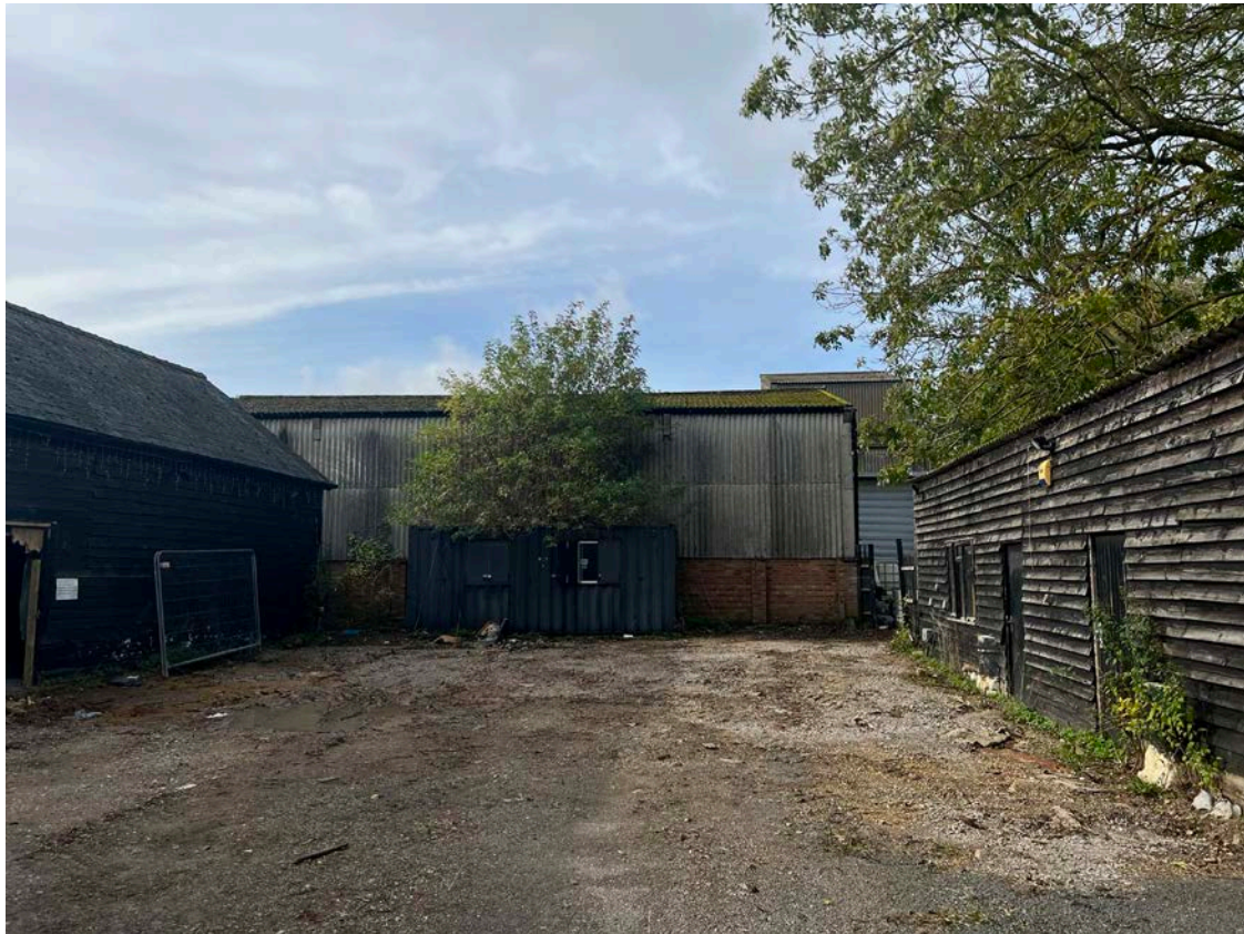
Historic barn - external views
