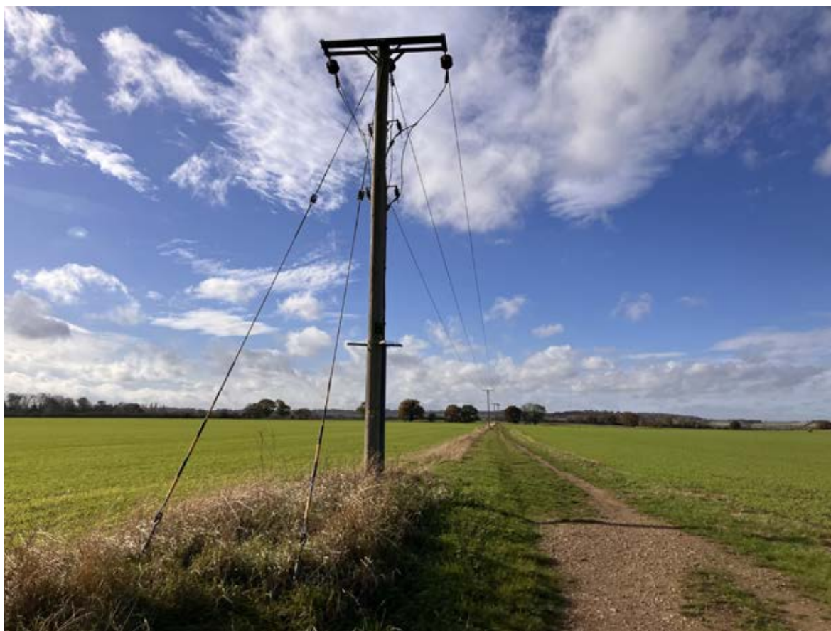
Plate 2: View looking west from Bedford Road along the PROW north from south eastern corner of the Site
