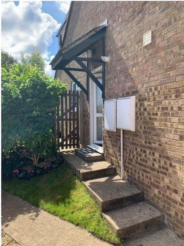
Existing entrance to side of house which will become entrance into proposed side extension.
