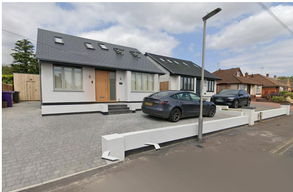
Figure 5: Nos 43 and 45 Manton Road
