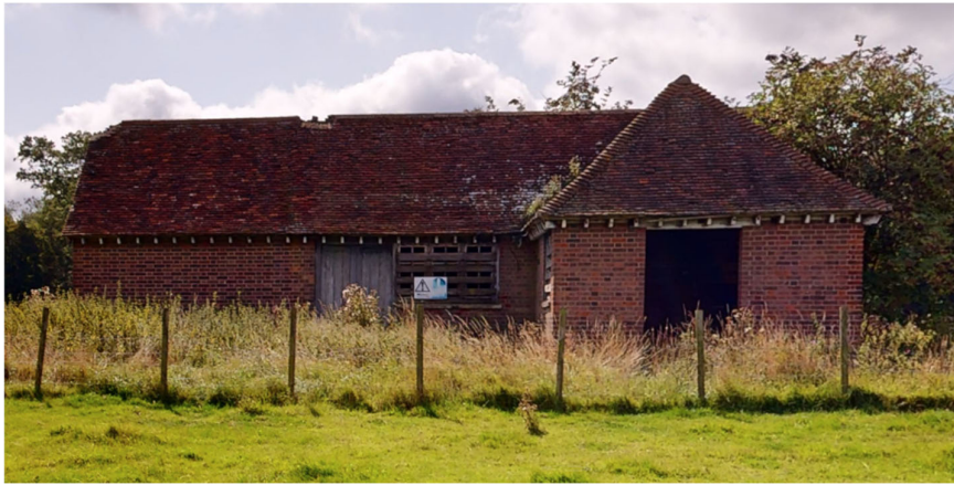
North Elevation of Pump House
